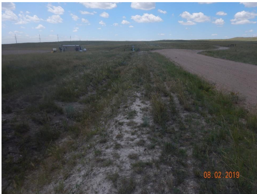
Photo 7: Photo taken from the north end of the location, facing west. Photo shows the perimeter stormwater ditch during initial construction activities remaining. Ditch does not appear to be needed and requires reclamation.
