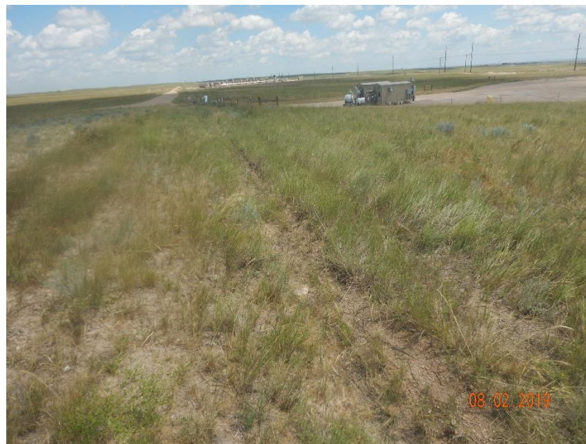
Photo 8: Photo taken from the north end of the location, facing east. Photo shows the perimeter stormwater ditch during initial construction activities remaining. Ditch does not appear to be needed and requires reclamation.
