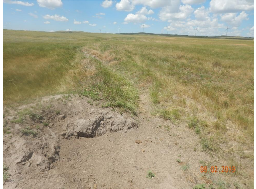
Photo 10: Photo taken from the south end of the location, facing northwest. Photo shows the perimeter stormwater ditch, and sediment during initial construction activities remaining. BMPs have not been maintained, do not appear to be needed and requires reclamation.
