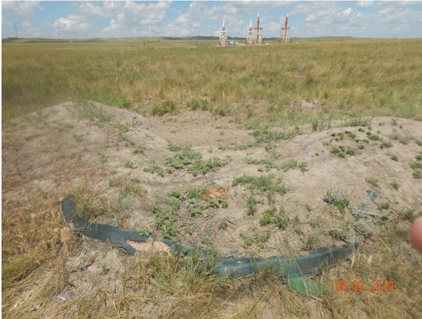
Photo 9: Photo taken from the south end of the location, facing north. Photo shows the perimeter stormwater ditch, and sediment during initial construction activities remaining. BMPs have not been maintained, do not appear to be needed and requires reclamation.
