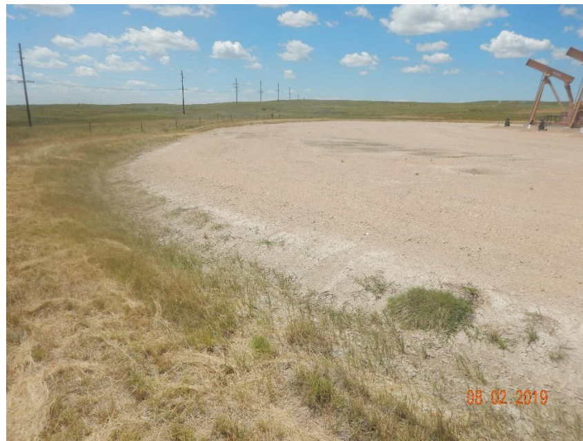
Photo 4: Photo taken from the southeast end of the location, facing west. Photos 1-3 provide an overview of the location from west, northwest to north. Photos show that only the areas of the access road, and immediate areas surrounding the wells appear to have been stabilized. Photo shows large areas that remain unstabilized where stormwater ponding outside of the perimeter ditch is evident.
