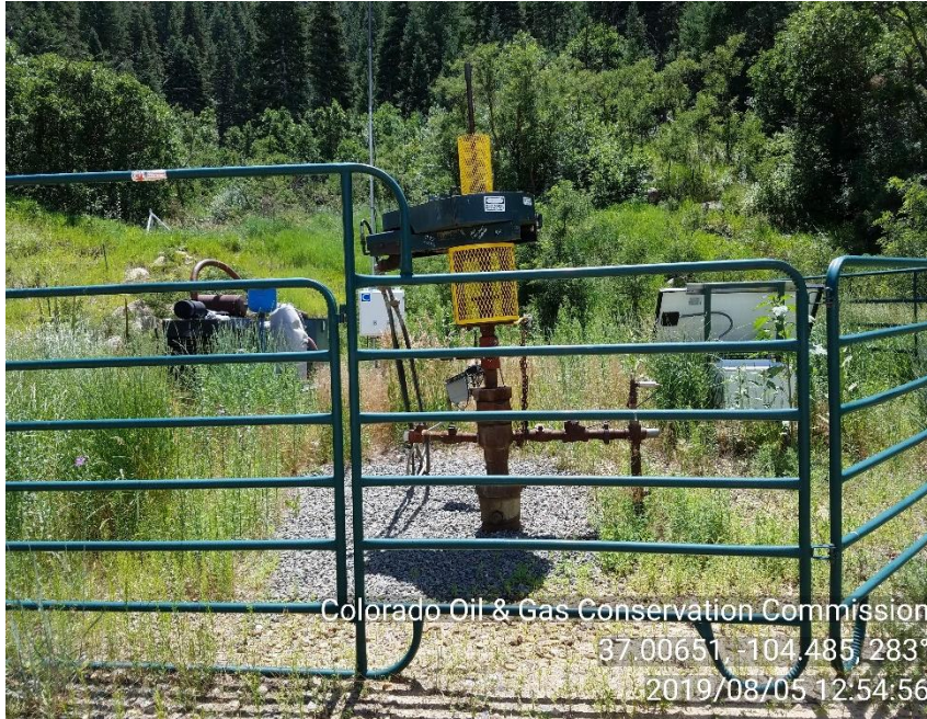
PHOTO 1: WELLHEAD/ WEED OVERGROWTH AROUND WELLHEAD AND ENGINE SKID. COMPLY WITH RULE 603. CA DATE 8-15-19
