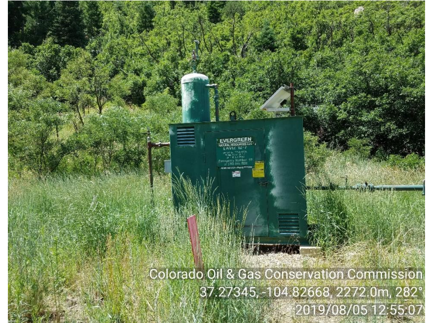
PHOTO 2: WELL SIGN/ WEED OVERGROWTH AROUND METER HOUSE. COMPLY WITH RULE 603. CA DATE 8-15-19
