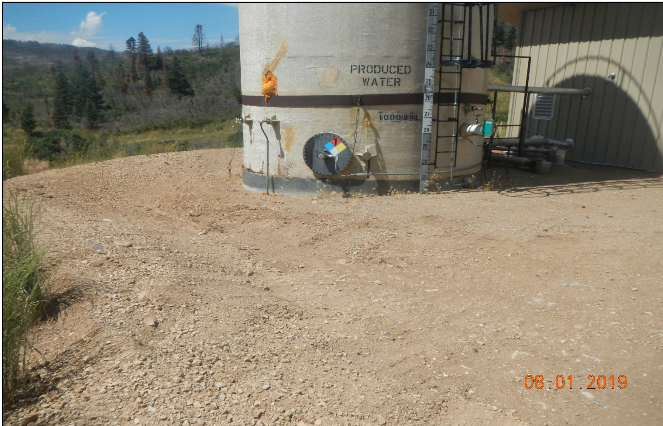
Photo 3. Facing toward the tank. Berm has been rebuilt.
