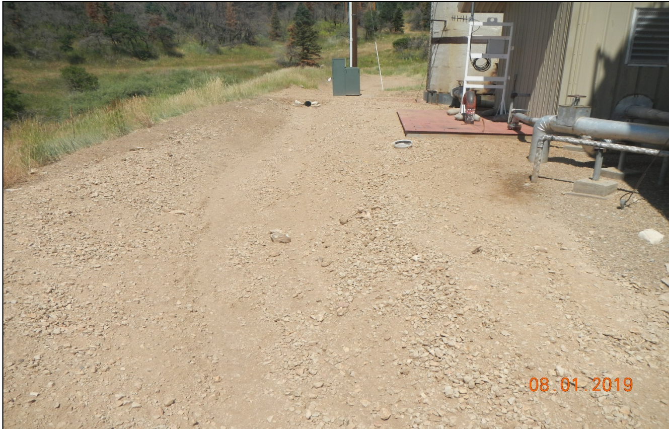
Photo 4. The contaminated soils behind the tanks have been removed and replaced with road base material.
