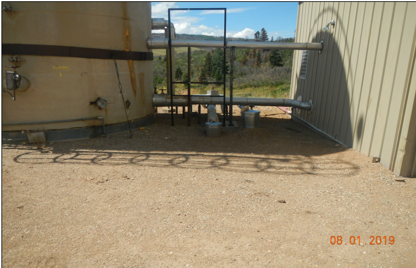
Photo 2. The secondary containment at discharge point has been repaired.
