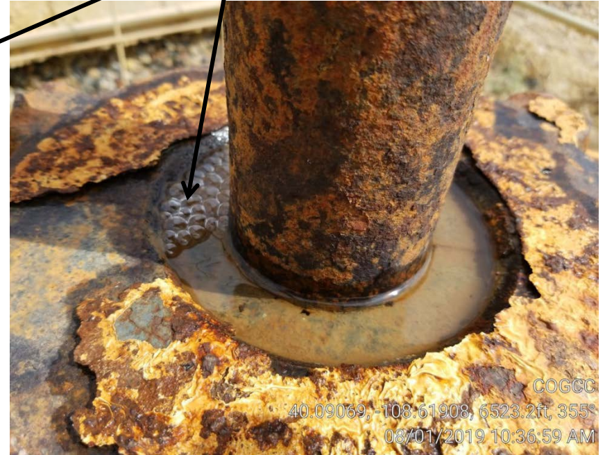
Photo 3. Gas leak.
