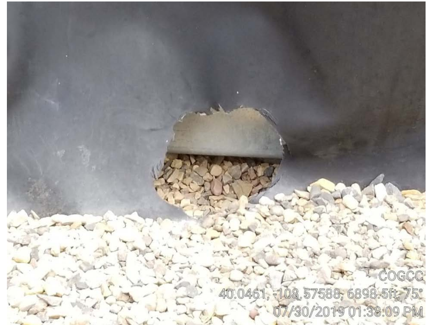
Photo 3. Tank liner hole.
