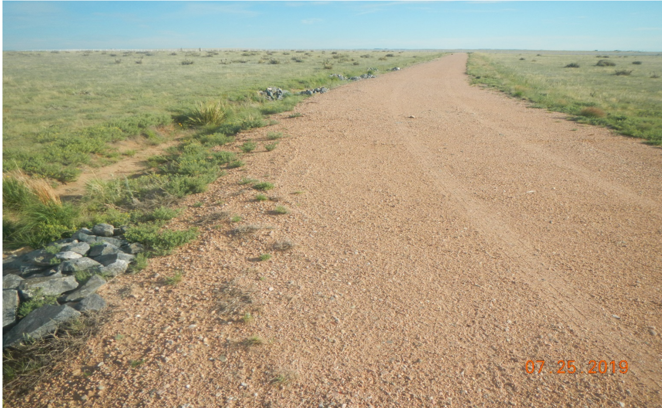
Photo 6. Rock check dams have been installed further up the road from the gate shown in photo 4. This photo depicts compliance of the corrective action.
