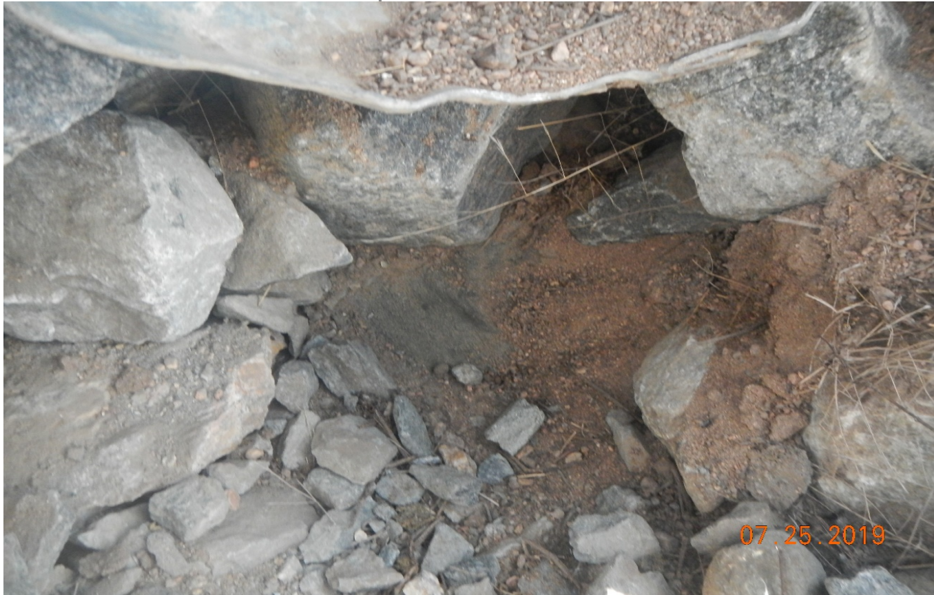
Photo 10. Geotextile was installed at the culverts outlet protection. This photo depicts compliance of the corrective action.
