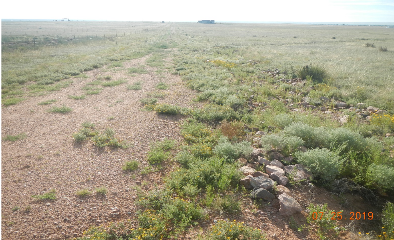
Photo 1. Facing east on the access road. Rock rip/rap can be seen in the drainage channel. There is desirable and undesirable weedy vegetation establishing in the drainage.
