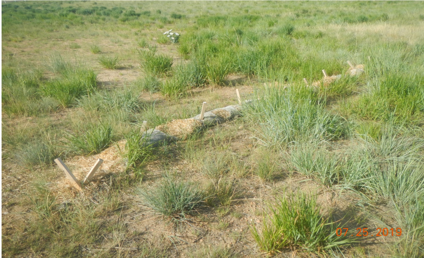
Photo 14. Wattles installed at the location have degraded and need to be removed or replaced.
