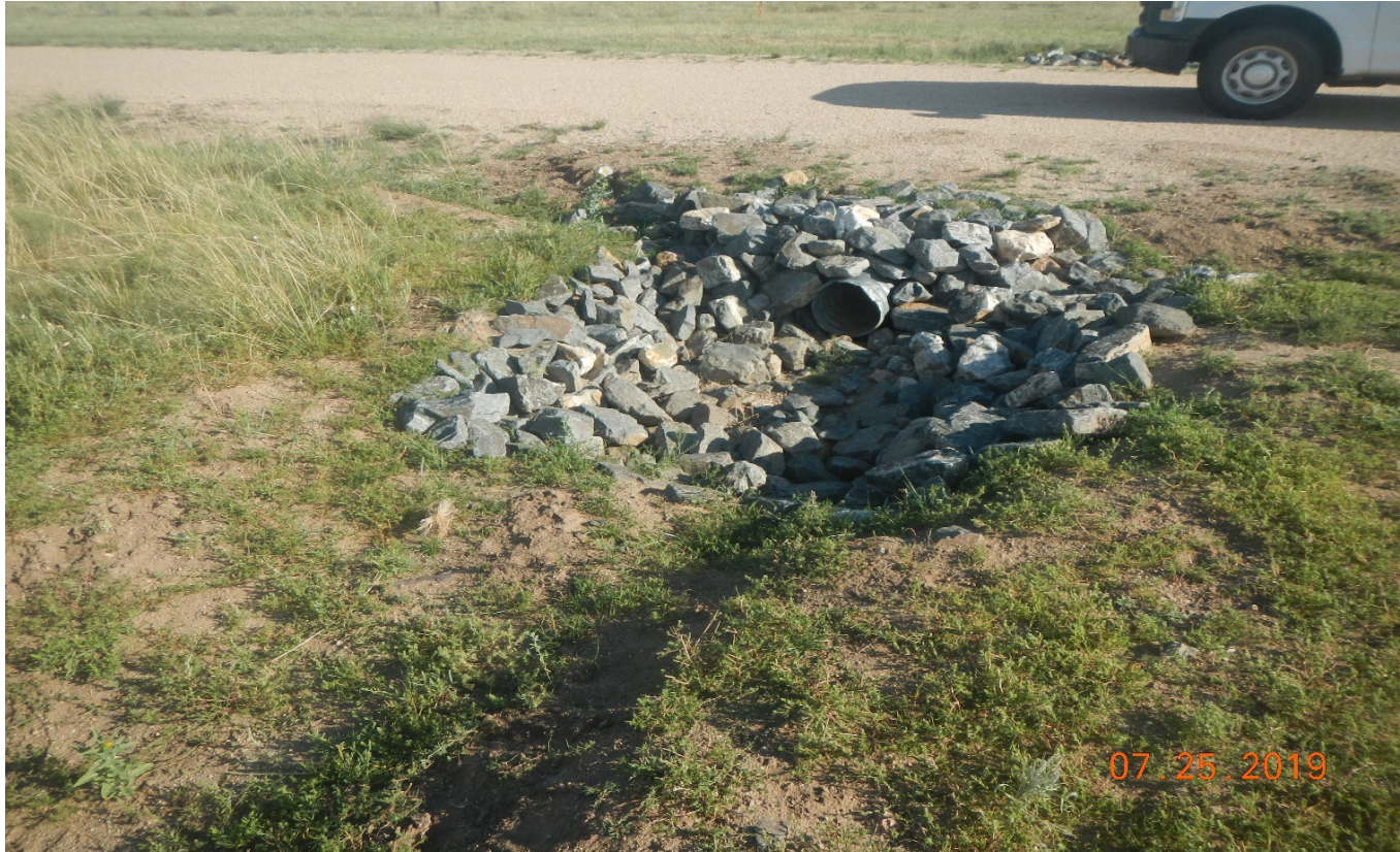
Photo 8. The outlet culvert rock rip/rap has been lowered to allow sediment to settle and not restrict stormwater flow. This photo depicts compliance of the corrective action. There is desirable and some undesirable weedy vegetation.
