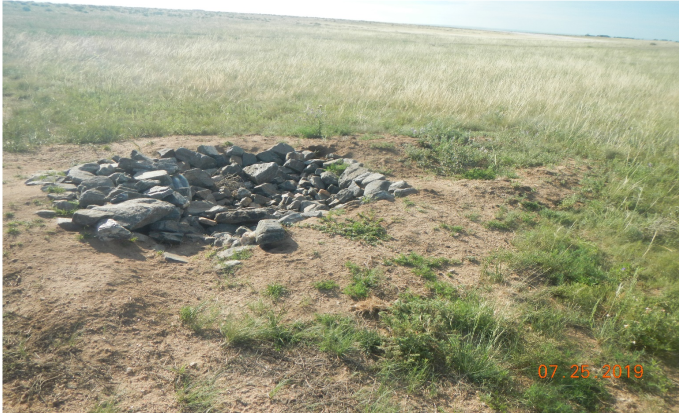
Photo 9. The outlet culvert rock rip/rap has been lowered to allow sediment to settle and not restrict stormwater flow. This photo depicts compliance of the corrective action.
