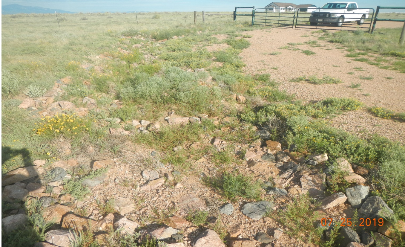
Photo 5. Rock rip/rap can be seen in the drainage channel. Rock check dams have been lowered to allow water flow. This photo depicts compliance of the corrective action. There is desirable and undesirable weedy vegetation establishing in the drainage.
