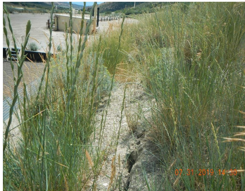
Subsidence of unstable cut slope behind tank battery.
