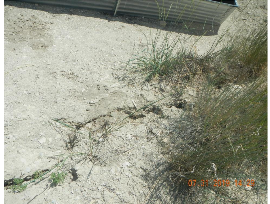
Subsidence of unstable cut slope behind tank battery.
