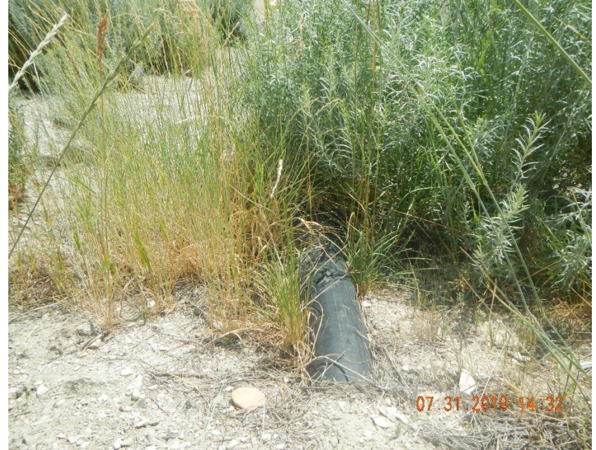
8" black poly line exposed at entrance near tank battery and the cut off end comes out on other the side of roadway and entrance.
