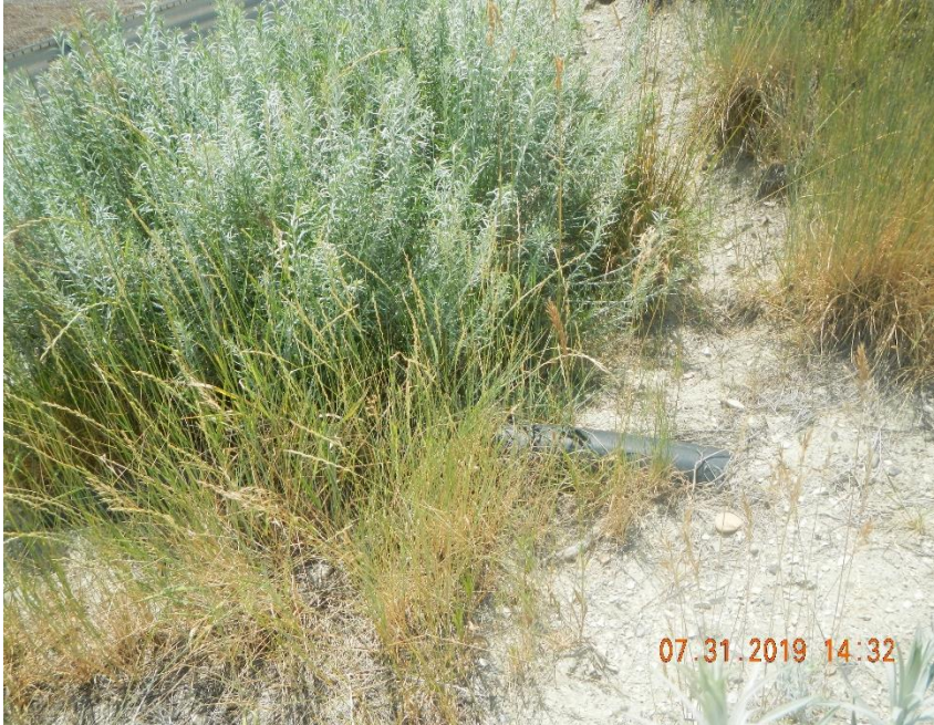
8" black poly line exposed at entrance near tank battery and the cut off end comes out on other the side of roadway and entrance.
