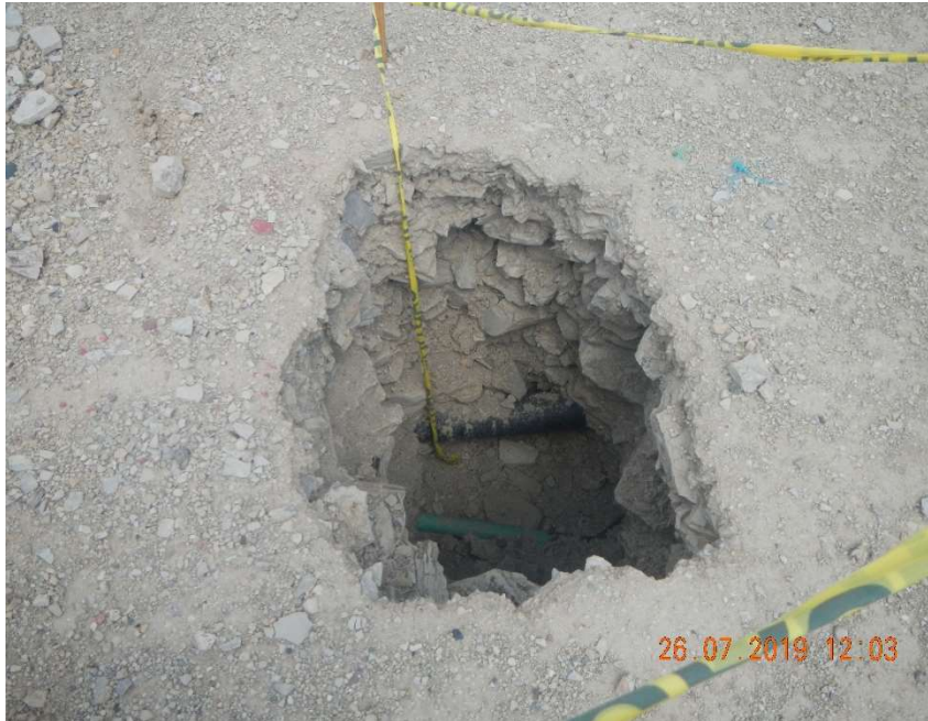
Photo #3 – View of the 3 feet by 4 feet by 6 feet deep excavation located southwest of the separators.
