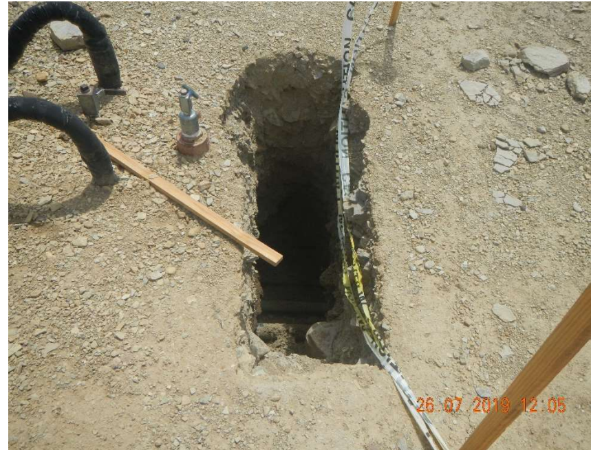
Photo #4 – View of the 1.5 feet by 4 feet by 6 feet deep excavation located southwest of the separators.
