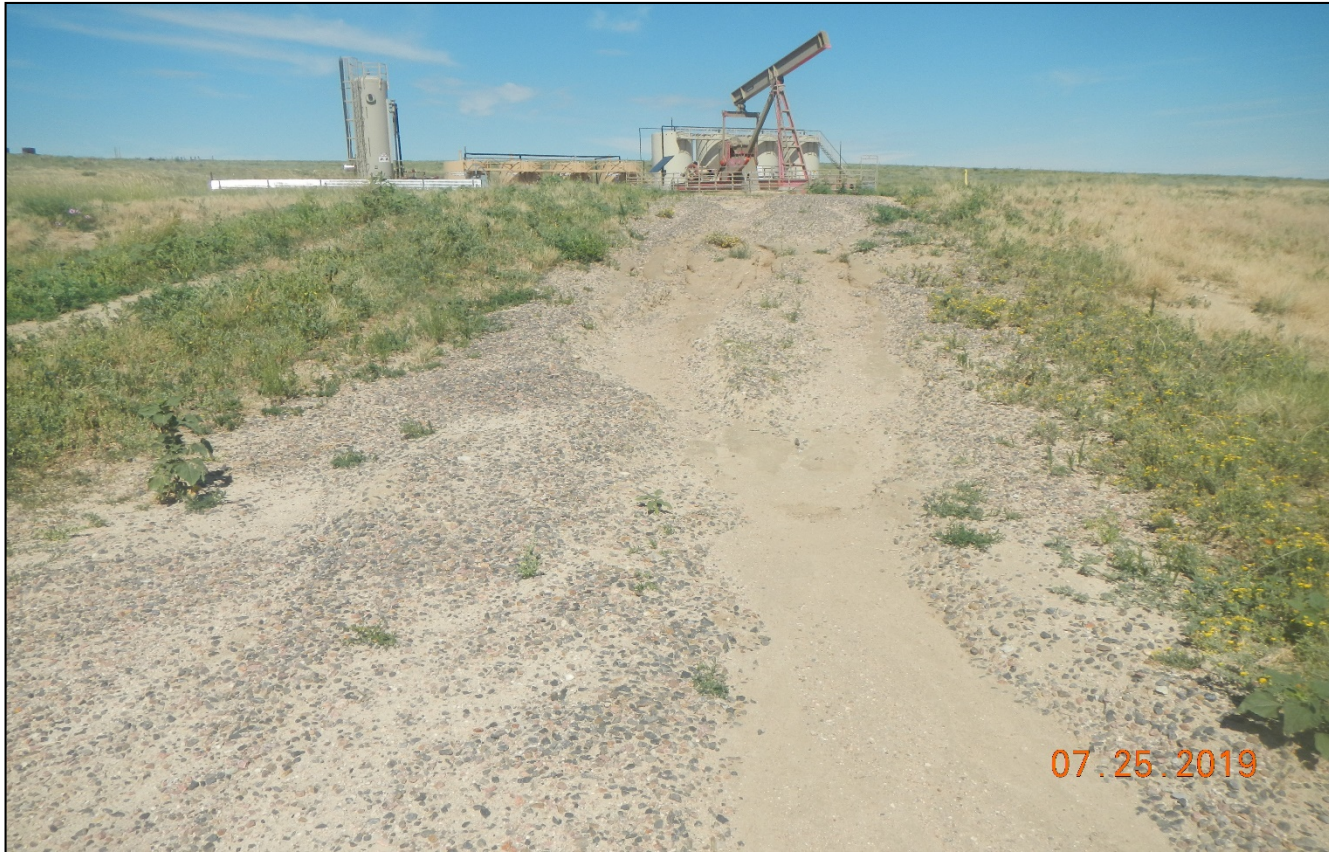
Photo 3. Facing northeast toward the location. There is erosion occurring along the access road.
