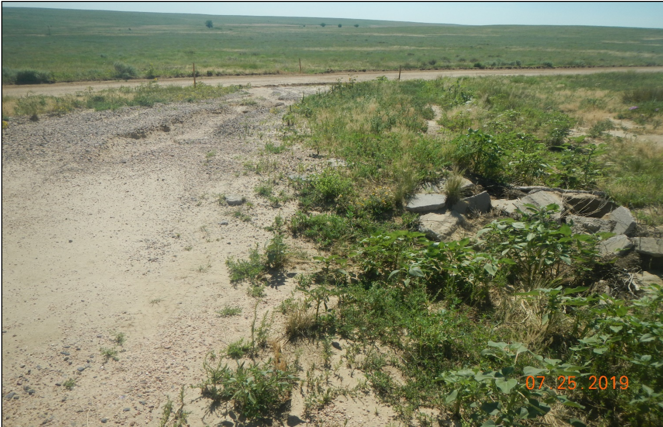
Photo 4. Facing back toward the access road. Rocks are piled in the drainage which is causing stormwater to flow down the access road.
