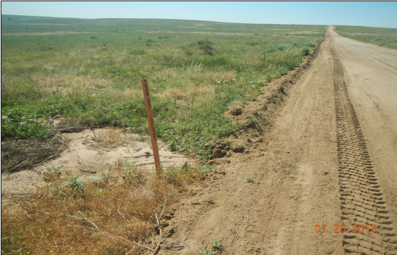
Photo 2. A culvert along the main road is filled in with sediment.
