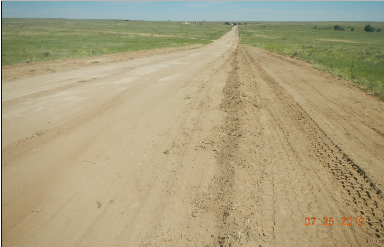
Photo 1. Facing north along the main road. The road was recently graded and widened. The side of the road was disturbed and needs to be revegetated.
