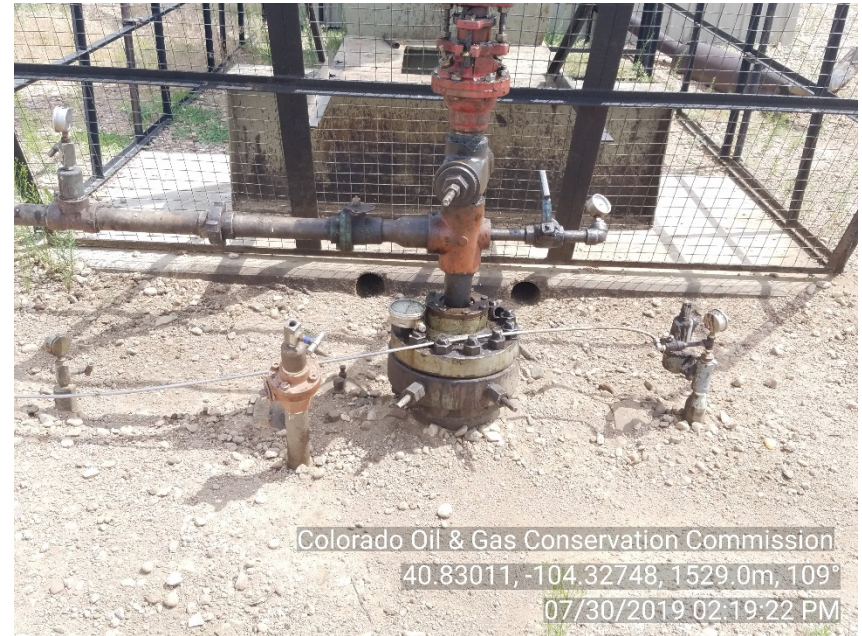
Photo #4 Smuggler 16-10-62 Battery Weeds & Stained soil appears mitigated Bradenhead NOW plumbed to surface
