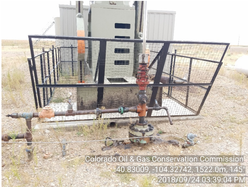
Photo #3 Smuggler 16-10-62 Wellsite Weeds, stained soil Bradenhead NOT plumbed to surface prior insp.
