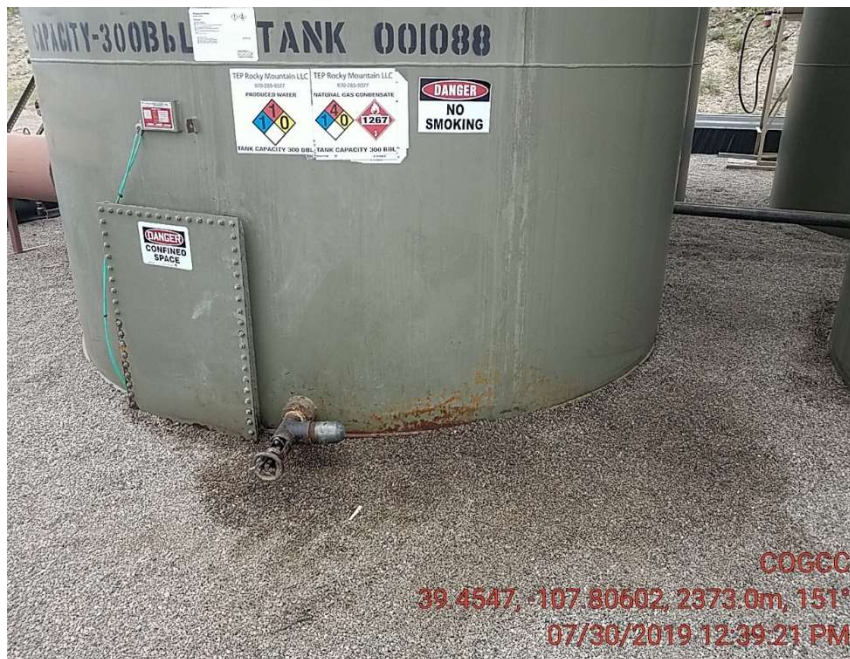
3 Staining next to tank valve
