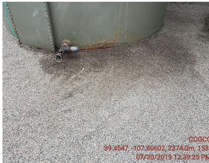
4 Staining next to tank valve
