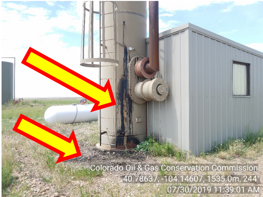
Photo #9 Birds of Prey 36-10-61 Treater Stained soil, equipment
