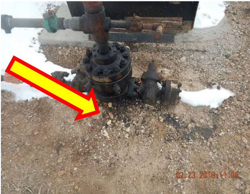
Photo #7 Birds of Prey 36-10-61 Wellhead Stained soil prior insp.
