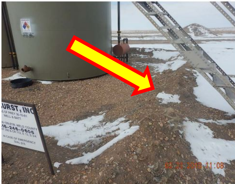
Photo #5 Birds of Prey 36-10-61 Tank Battery Low berms prior insp.
