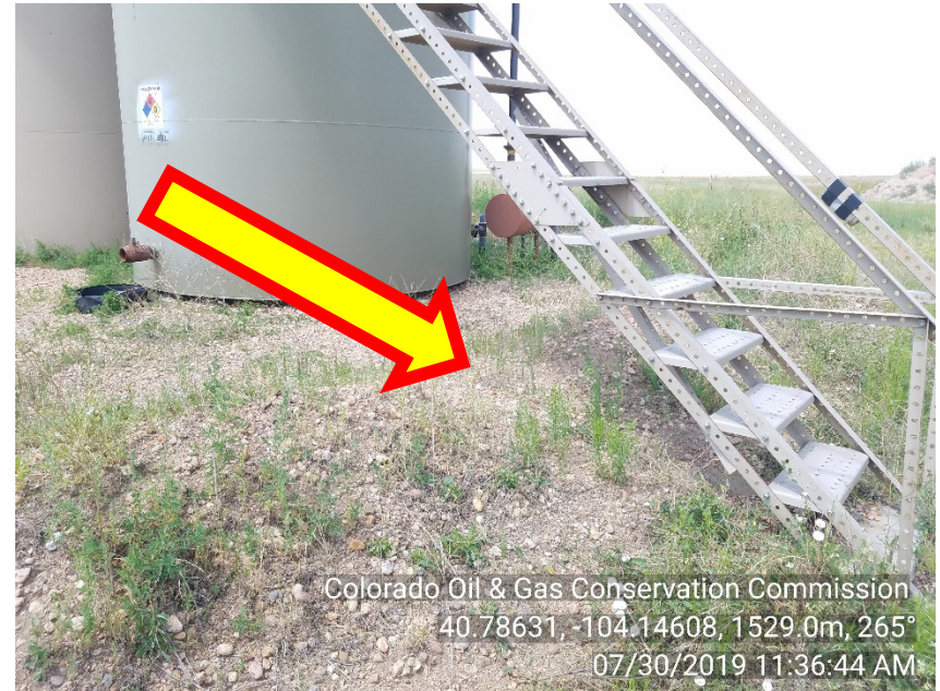
Photo #6 Birds of Prey 36-10-61 Tank Battery Low berms – NOT addressed
