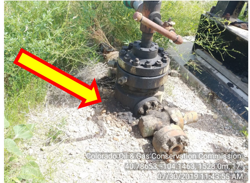
Photo #8 Birds of Prey 36-10-61 Wellhead Stained soil – NOT addressed
