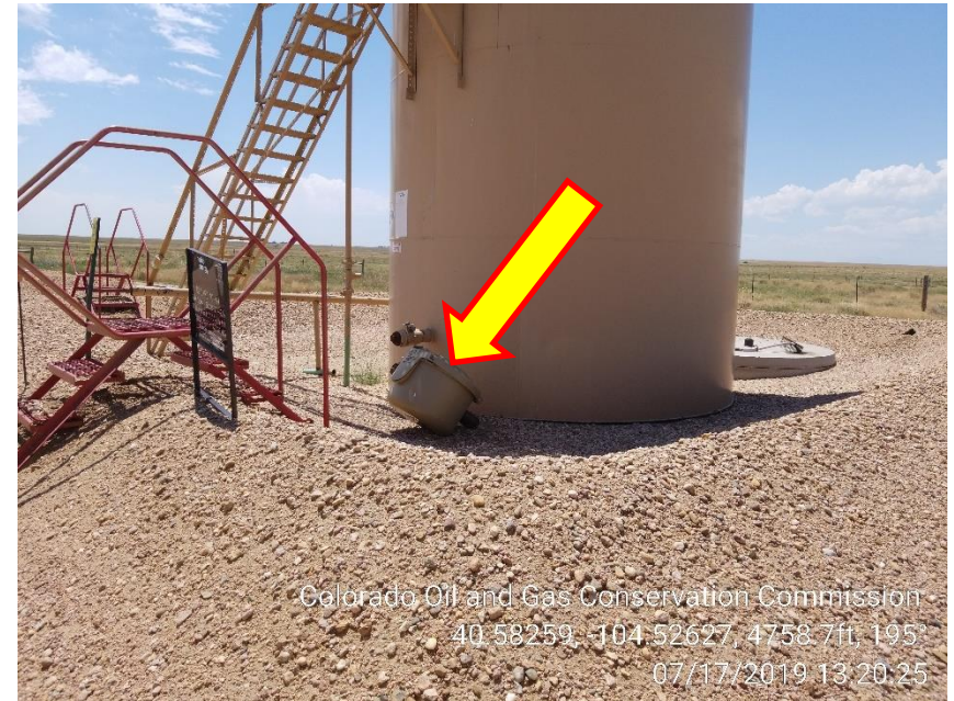
Photo 4 – Unused Loadline Bucket inside Tank berm
