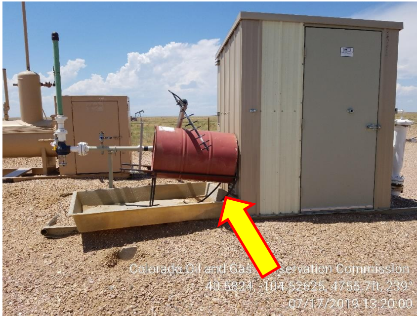
Photo 3 – Unused Methanol Tank and Containment
