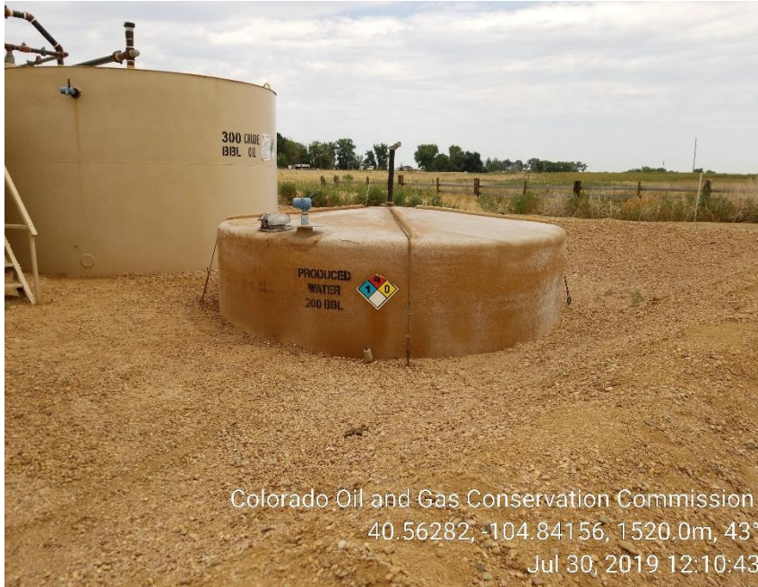
Photo 3: Labeling on produced water tank added
