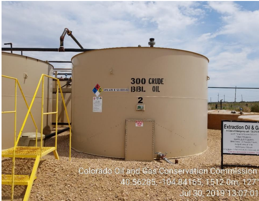
Photo 5: Labeling added to crude oil tank
