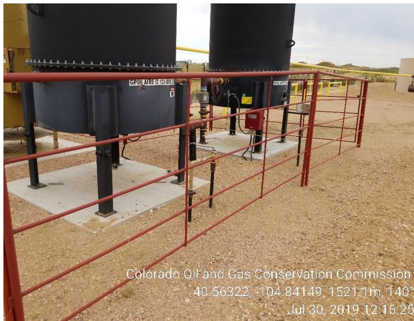
Photo 7: Risers removed
