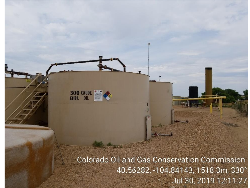
Photo 4: Labeling added to crude oil tank
