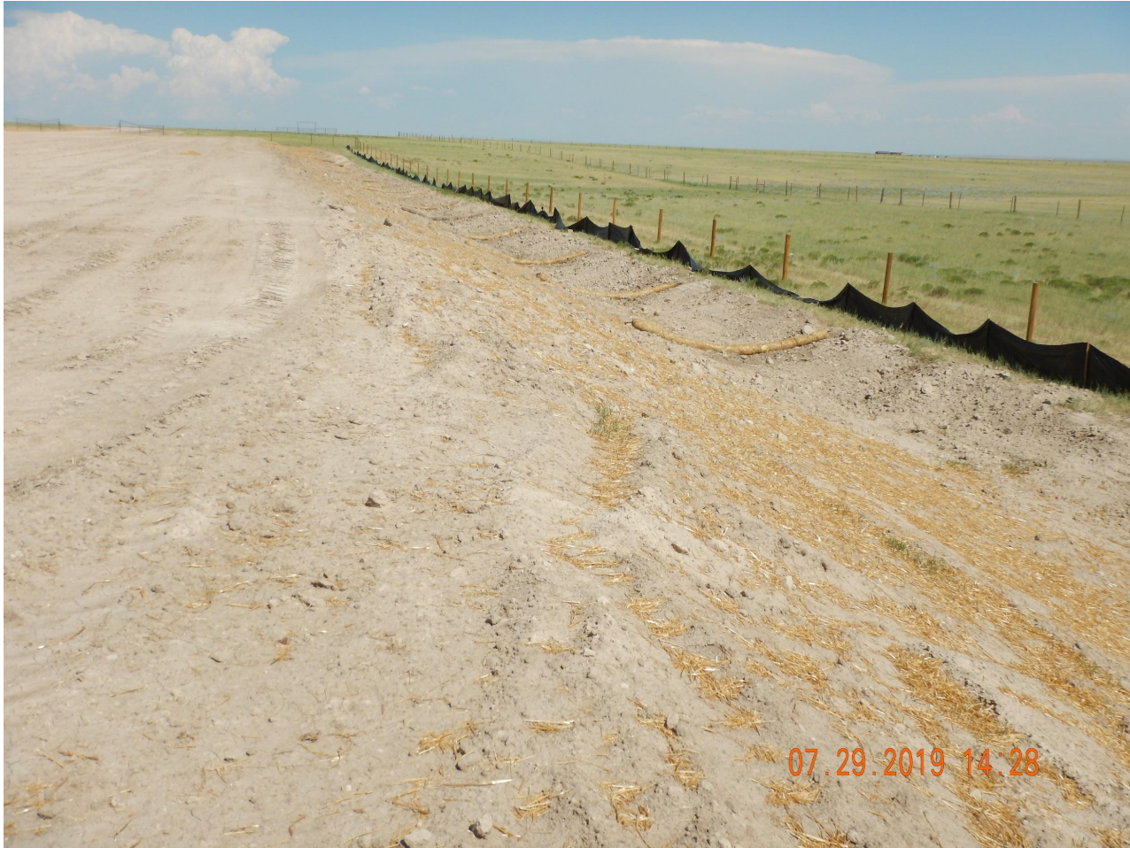
Photo 3. Photo taken from the southwestern location, facing East. Operator has installed straw wattles along portions of the ditch. Portions of the ditch may need to be
