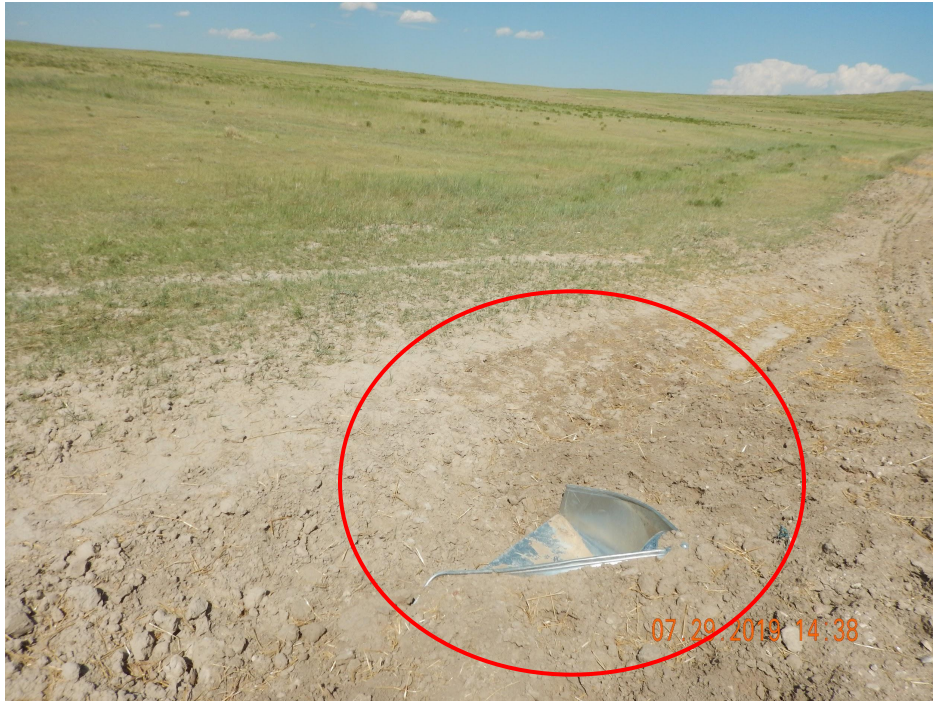
Photo 9. Photo taken from a portion of the access road, facing East. Photo illustrates inlet and outlets of culverts still need to be stabilized.
