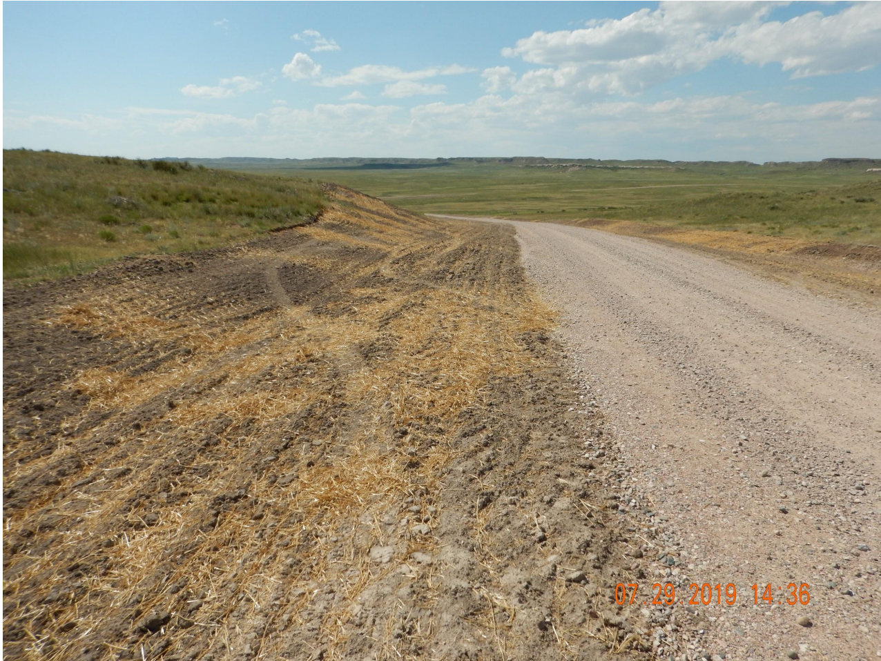
Photo 8. Photo taken from a portion of the access road, facing Northwest. Access road was pre-existing. Operator has seeded along the roadside ditch. Mulch does not appear to have been installed evenly which may not protect the seeded soil.
