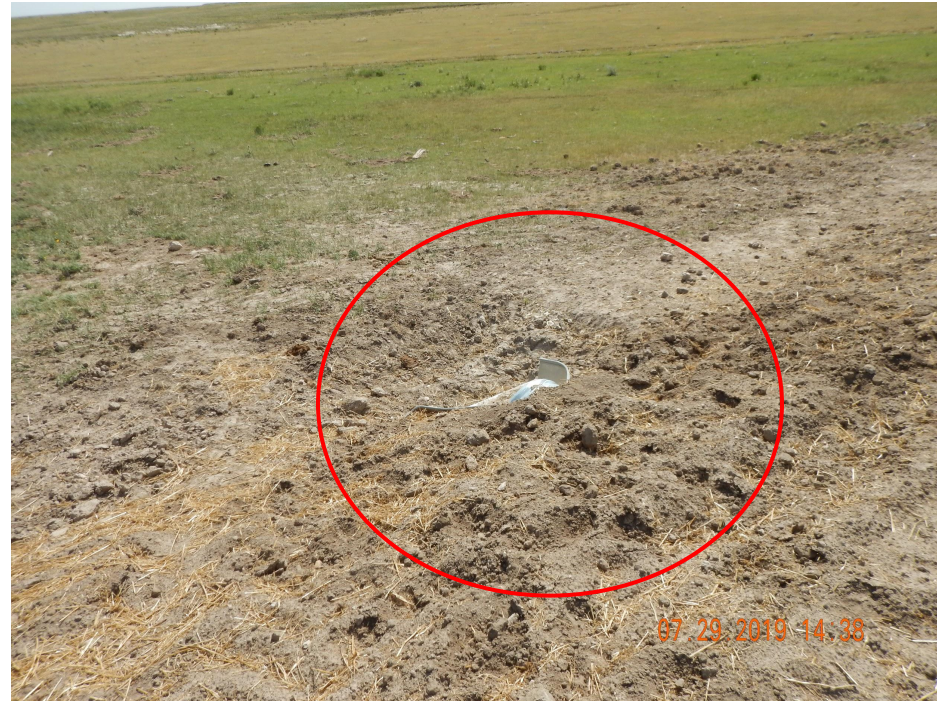
Photo 10. Photo taken from a portion of the access road, facing East. Photo illustrates inlet and outlets of culverts still need to be stabilized.
