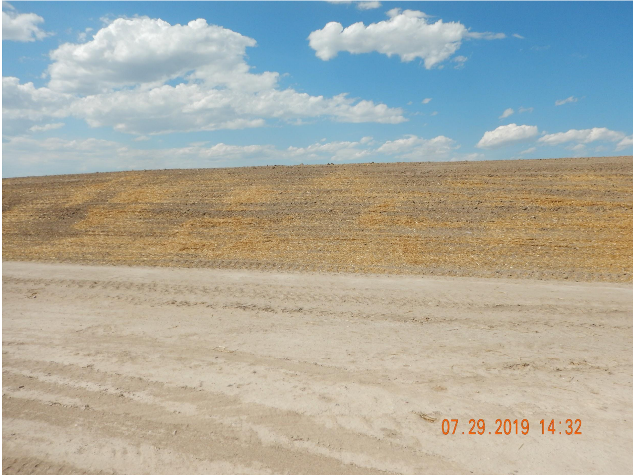
Photo 6. Photo taken from the northern location, facing North. Photo illustrates the topsoil stockpile which has been seeded and mulched.
