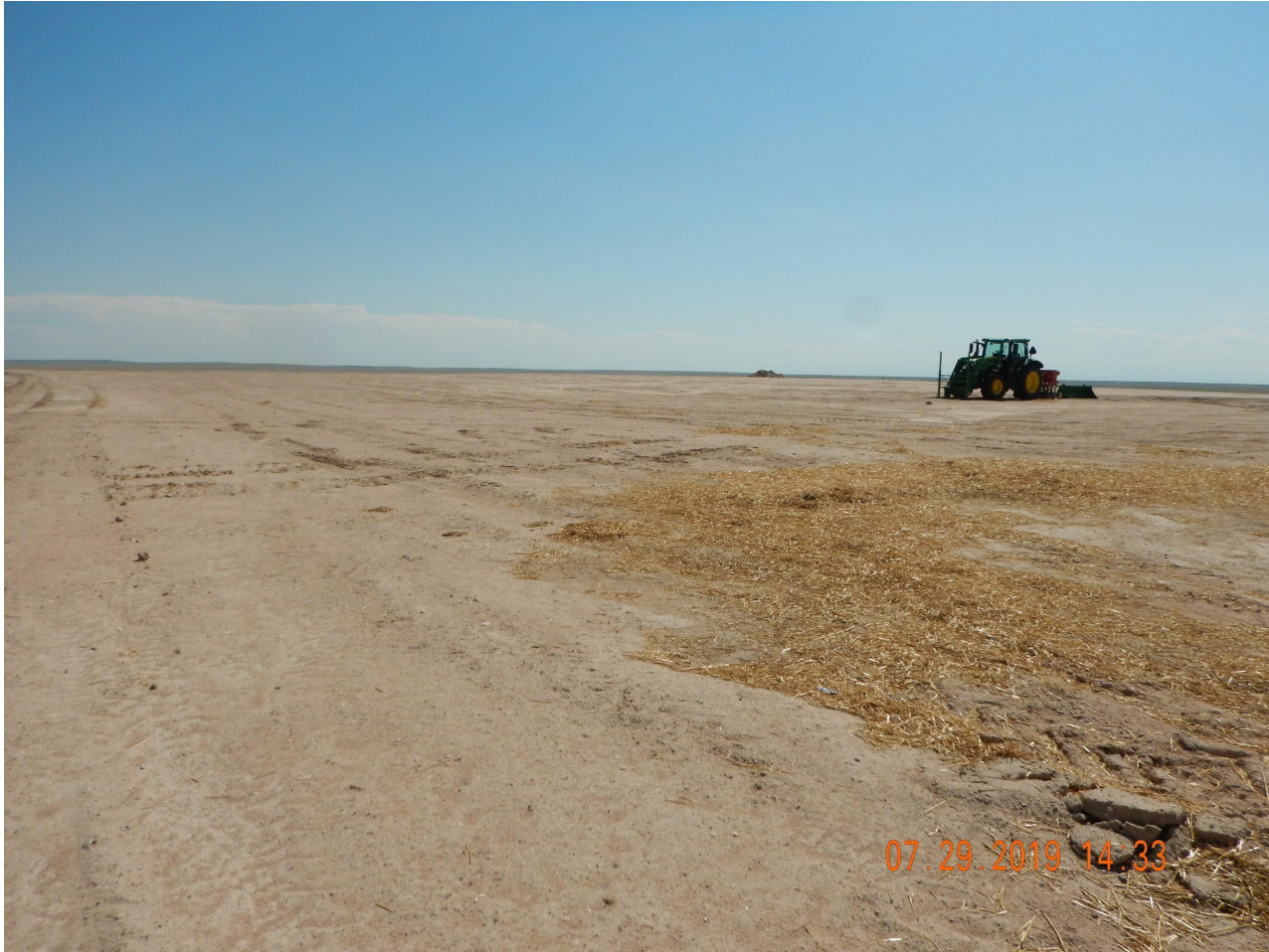
Photo 7. Photo taken from the northeastern location, facing South. Photo illustrates other portions beyond the well locations has only been compacted. Compaction alone may not be sufficient to properly stabilize the well pad from wind and water erosion.
