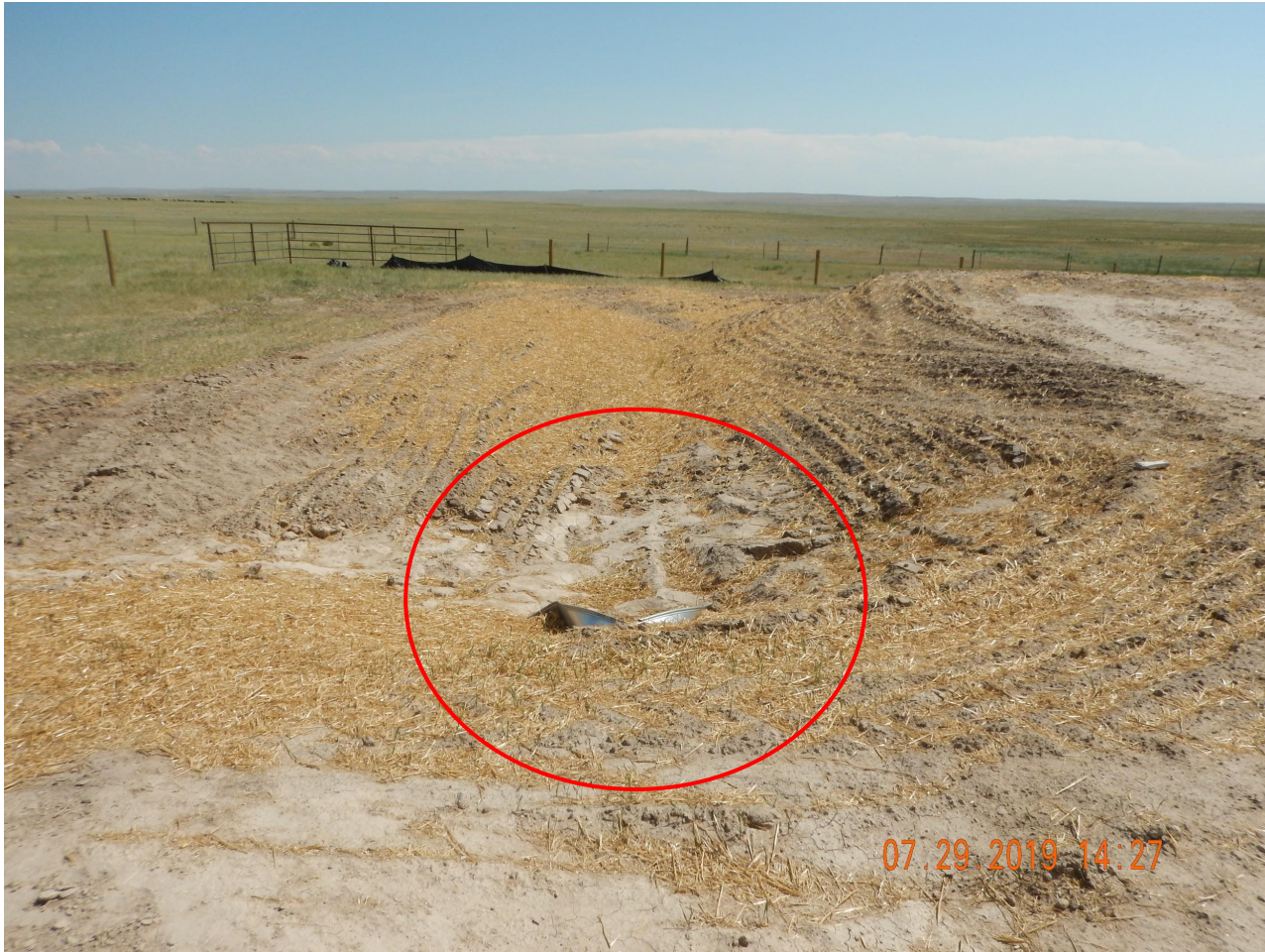
Photo 1. Photo taken from the entrance of the location, facing South. Operator has installed a ditch which is directed to a retention area. Ditch area has been seeded and mulched. Inlet and outlets of culverts still need to be stabilized. Silt fence BMP was used as the initial stormwater BMP and will be removed.
