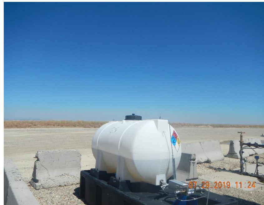
Chemical container at wells is missing label.
