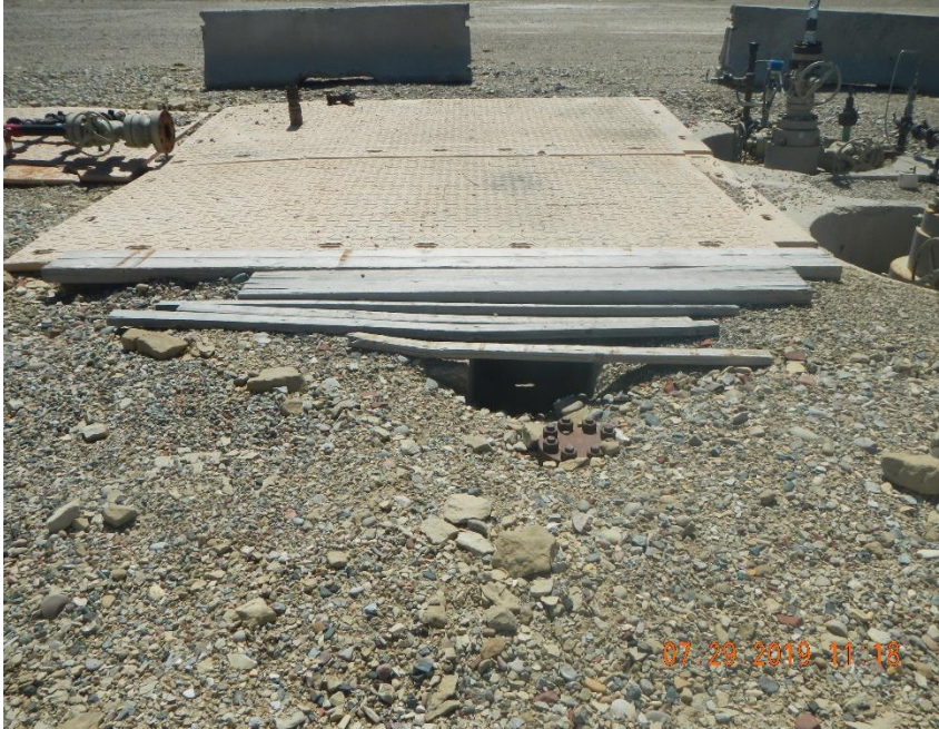
Cement cellar is not covered fully
