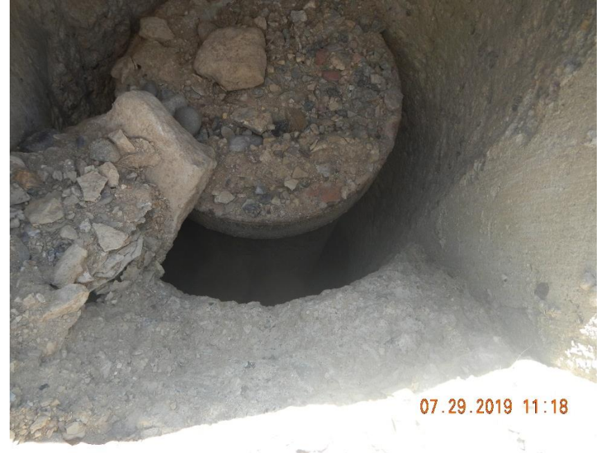
Rat hole has a void between casing and hole.
