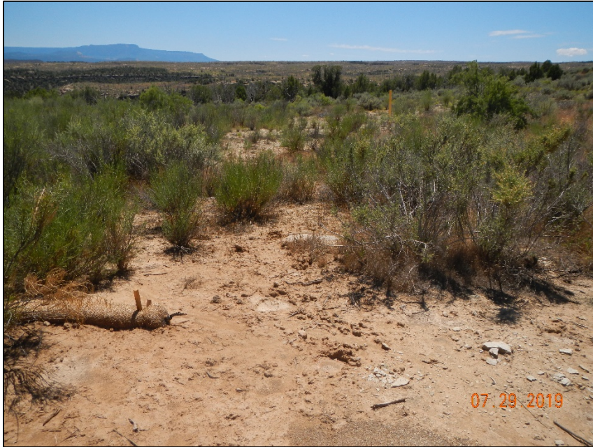
Photo #11 Photo of BMP that was recently put in place, allows erosions sediment to move around the waddle, letting sediment move south off location, choking out vegetation.
