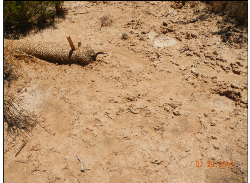
Photo #12 Photo of BMP that was recently put in place to stop erosion, allows erosions sediment to move around the waddle, letting sediment move south off location, choking out vegetation.
