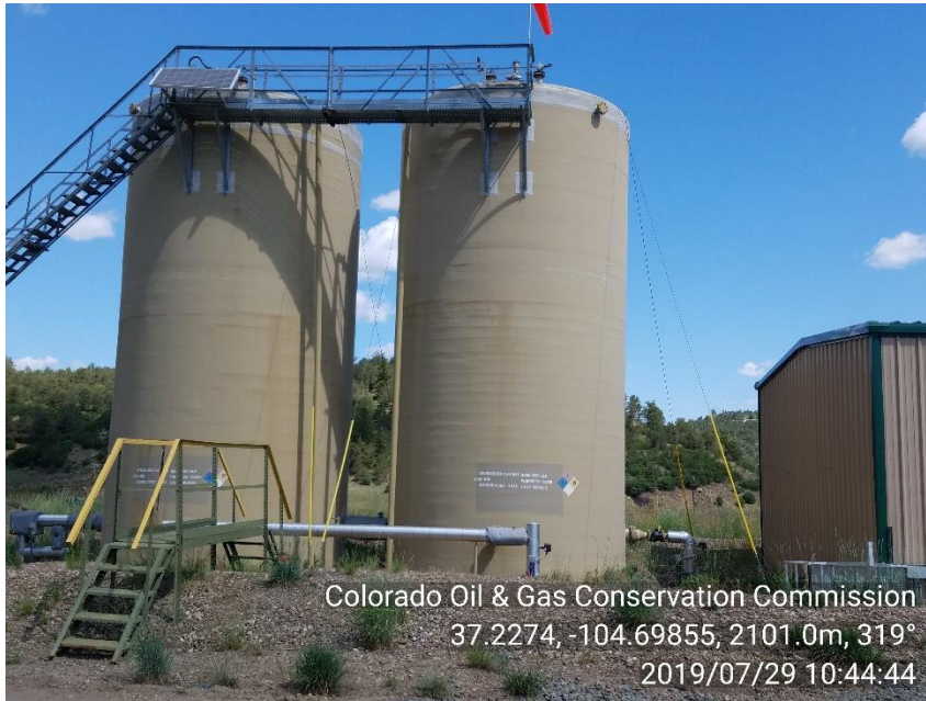
PHOTO 1: TANK BATTERY
