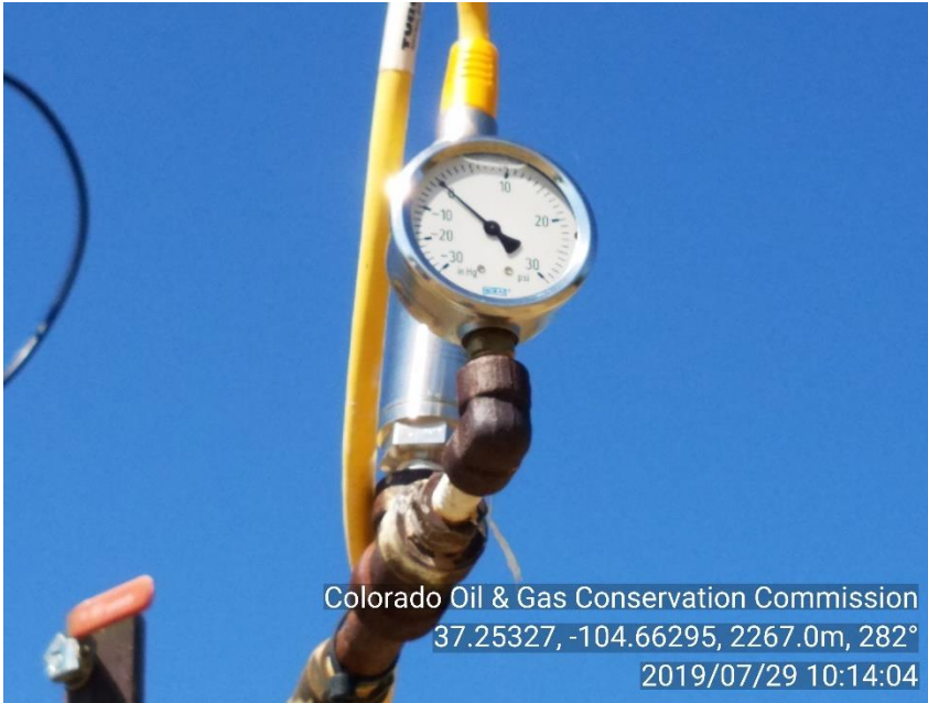
PHOTO 3: WELL IS SHUT IN 0 PSI ON INJECTION
