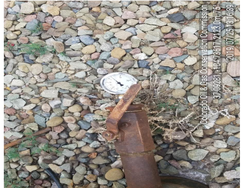
PHOTO 6: BRADEHEAD 3 PSI BLEW DOWN 3 PSI MONITORED FOR FLOW FOR 15 MIN. NO FLOW
