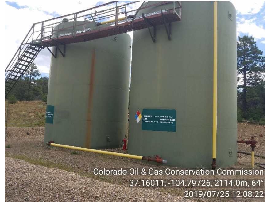
PHOTO 2: TANK BATTERY
