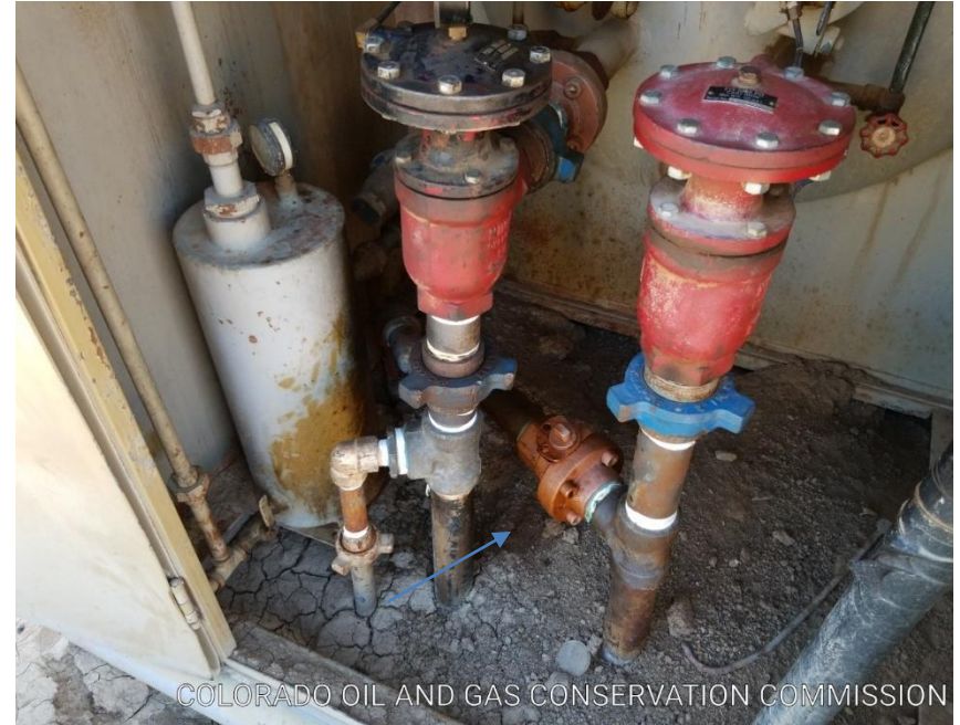
Pic 8 stained soil/mechanical issue in separator house
