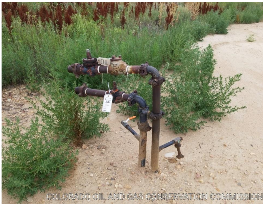
Pic 9 uncapped risers/possible leak
