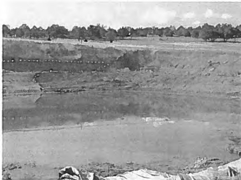
Torn pit liner of evaporation pond.
