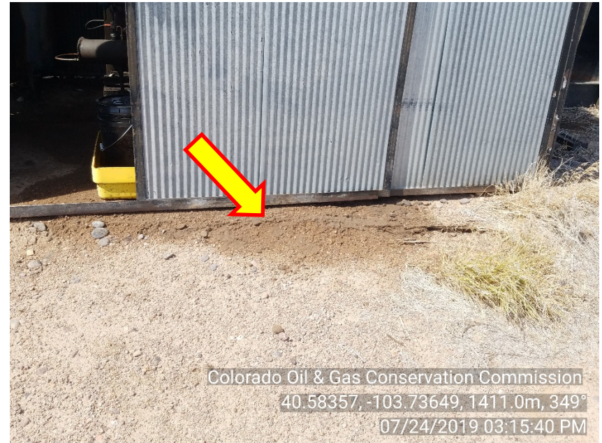
Photo #4 Henderson 1 Engine shed Stained soil - Outside
