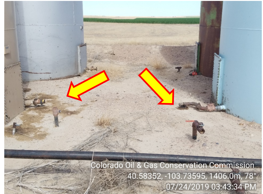
Photo #14 Henderson 1 Crude oil tanks Stained soil behind tanks remains
