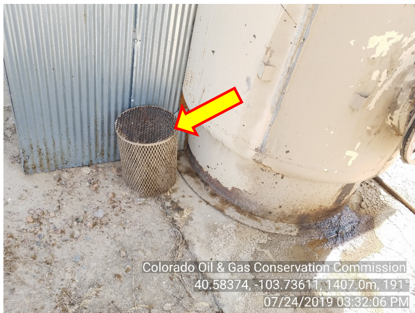
Photo #21 Henderson 1 West treater Bird protection device NOT on stack
