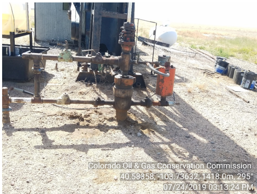
Photo #1 Henderson 1 (05-123-21201) Wellsite Bradenhead NOT plumbed to surface Stained soil
