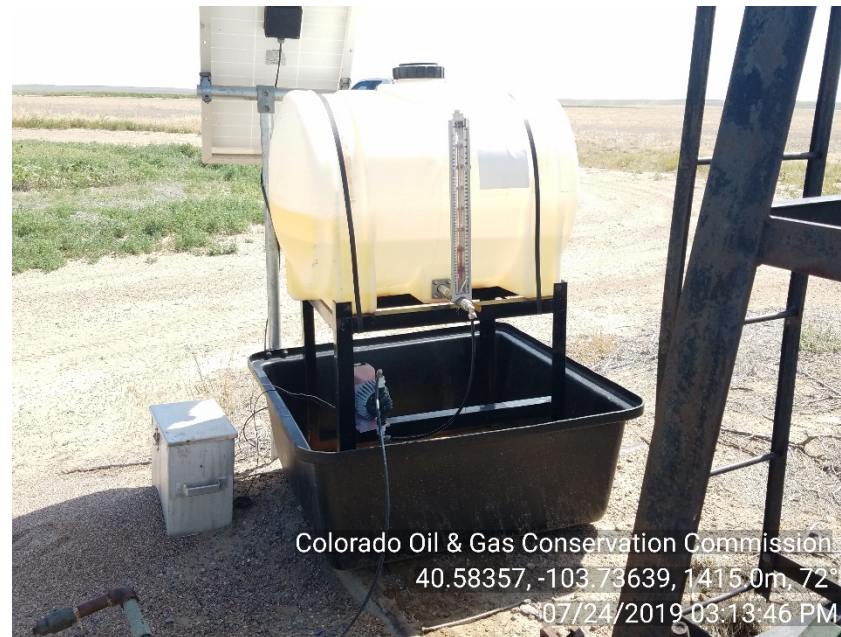
Photo #10 Henderson 1 Pumpjack Chemical pump tank NO legible contents / hazard label posted
