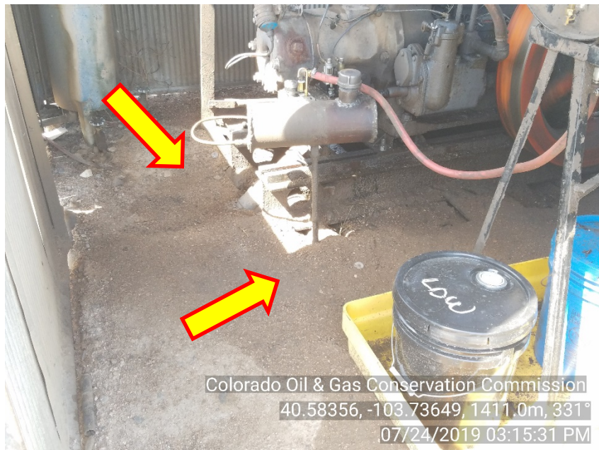
Photo #7 Henderson 1 Engine shed Stained soil - Inside
