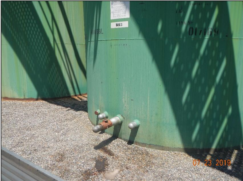
Photo #7 stained gravel inside tank containment
