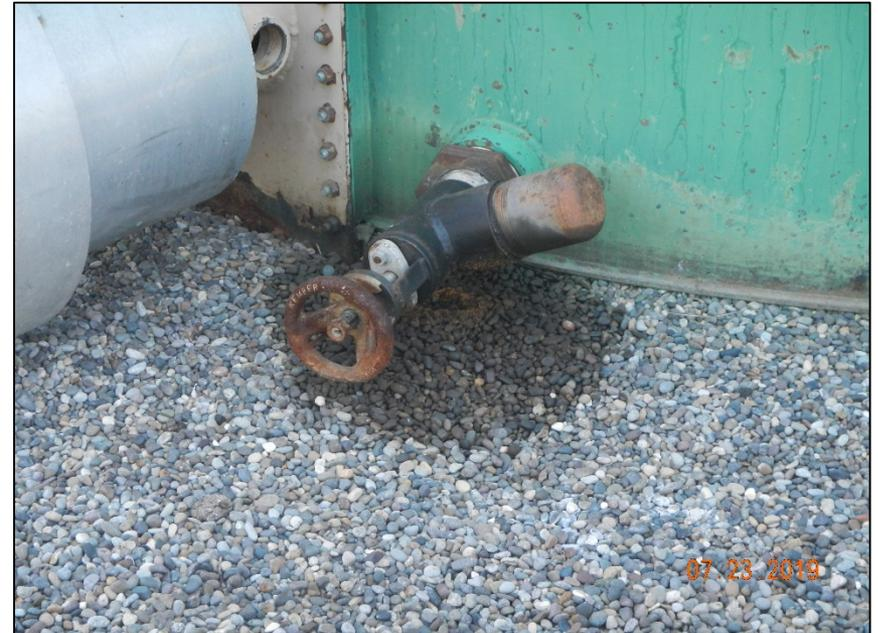
Photo #6 stained gravel inside tank containment
