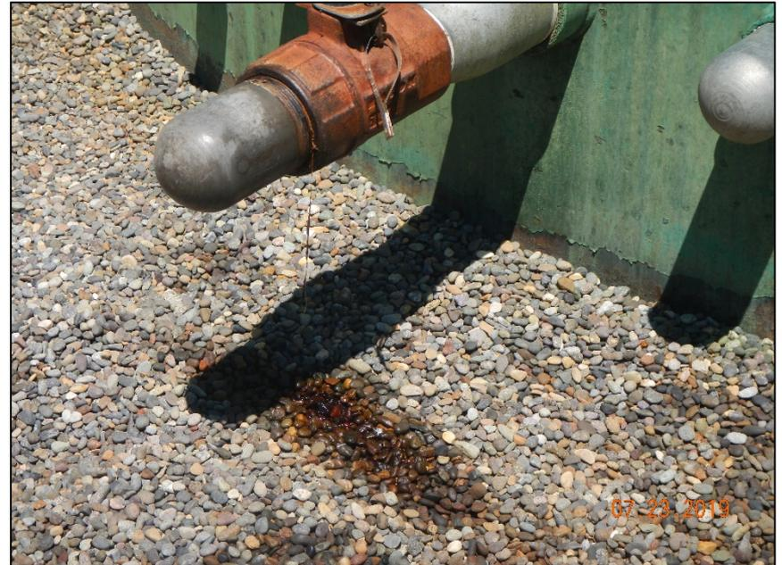
Photo #8 stained gravel inside tank containment
