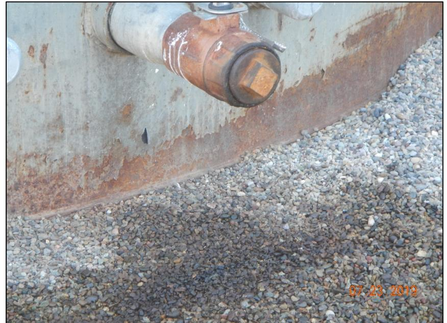
Photo #5 stained gravel inside tank containment
