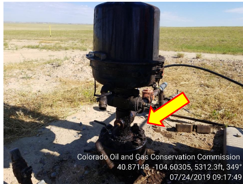
Photo 8 – Wellhead appears to be leaking,
