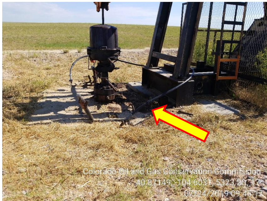
Photo 7 – Stained Soil at Wellhead
