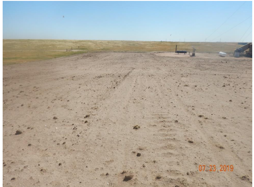
Photo 6: Photo taken from the northwest end of the location, facing east. Photo show soils have been replaced and location recontoured/regraded. However, unable to find evidence that location has had revegetation/reseeding activities conducted.
