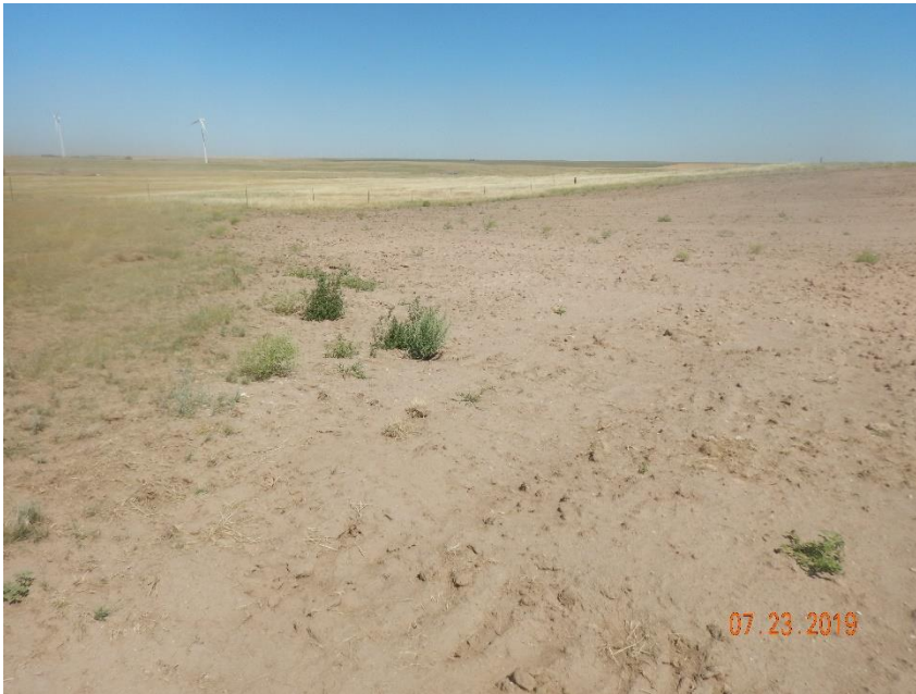
Photo 5: Photo taken from the southwest corner of the location, facing northwest. Photo show soils have been replaced and location recontoured/regraded. However, unable to find evidence that location has had revegetation/reseeding activities conducted.
