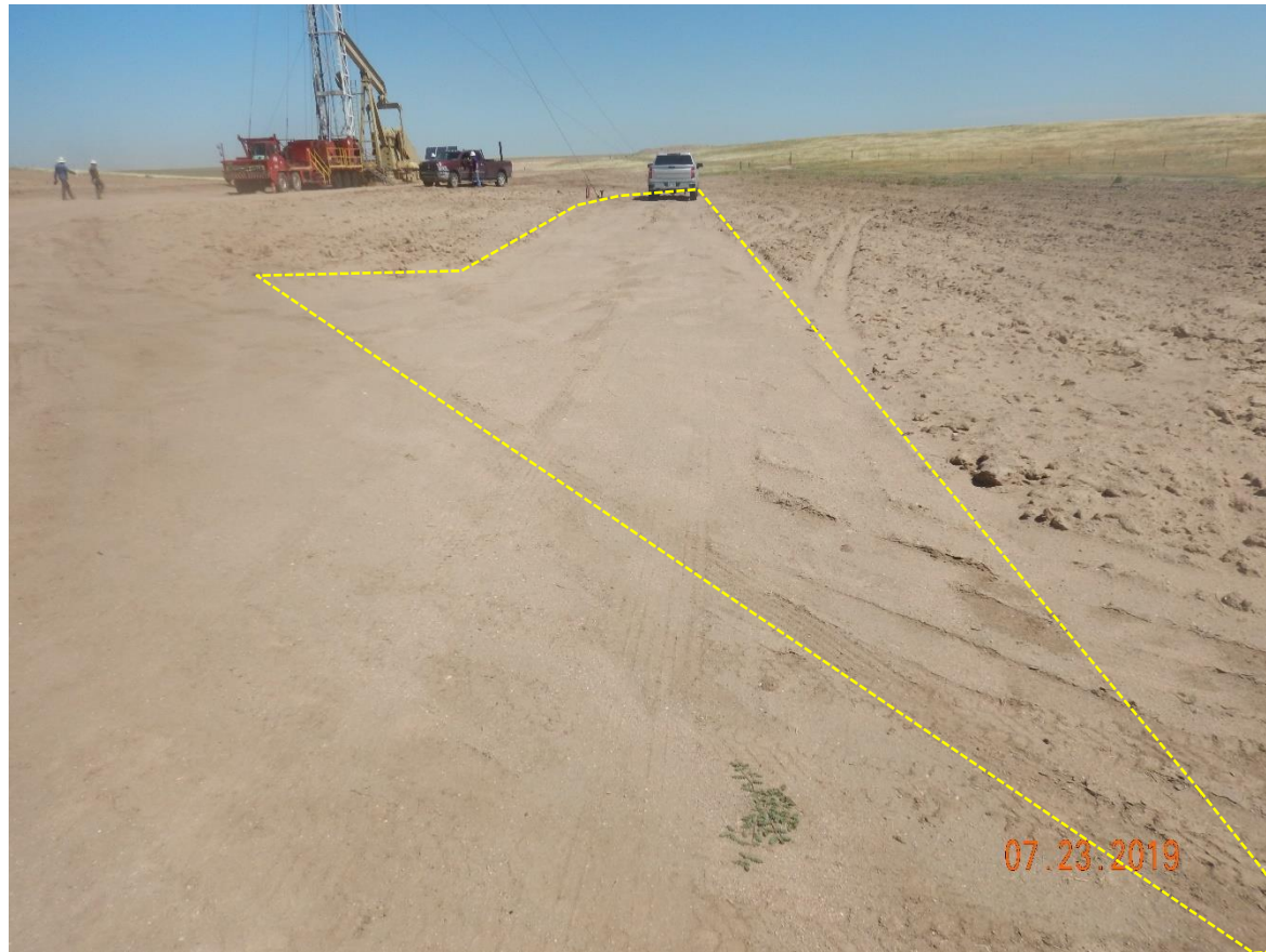
Photo 7: Photo taken from the location, facing north. Photo shows vehicle/equipment travel has re-disturbed the interim areas
