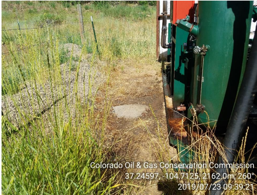
PHOTO 5: AREA OF IMPACTED SOIL APPEARS TO BE OIL FROM COMPRESSOR. Remove and dispose impacted material in approved manner, service and maintain equipment and self inspect to prevent recurrence of conditions per 1002.f(2) and 907. CA DATE 8-23-19
