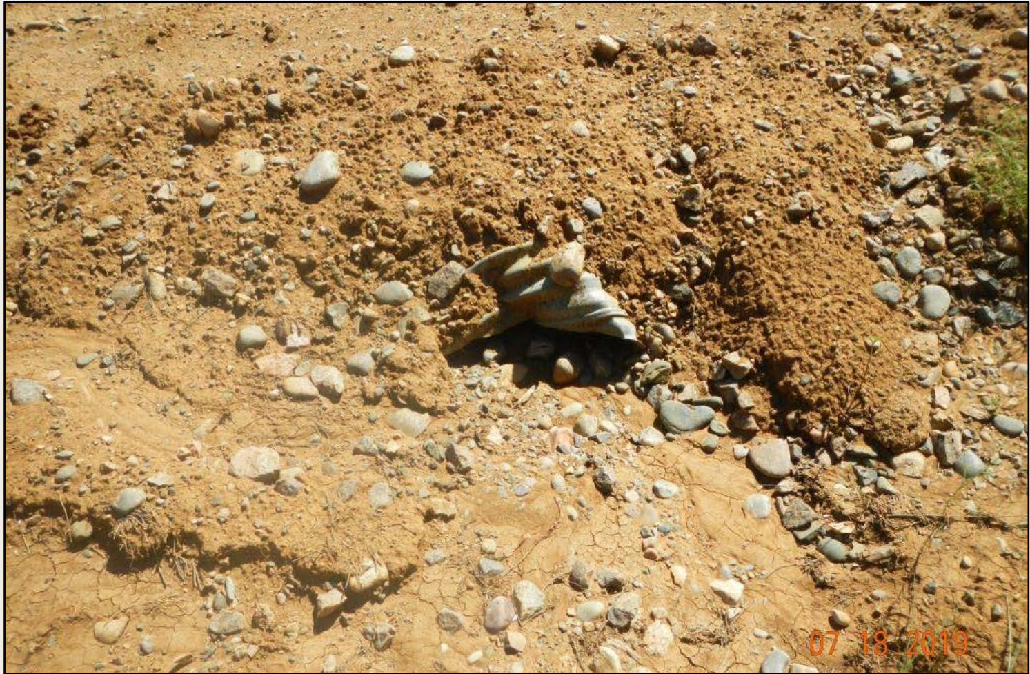
Photo 3. View of damaged culvert full of sediment and erosional rilling around culvert near the well pad entrance.
