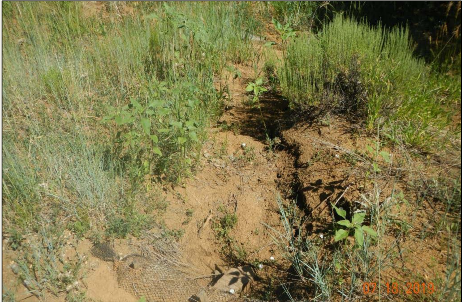
Photo 2. View of wattle full of sediment and erosional down-cutting downstream from culvert near well pad entrance.
