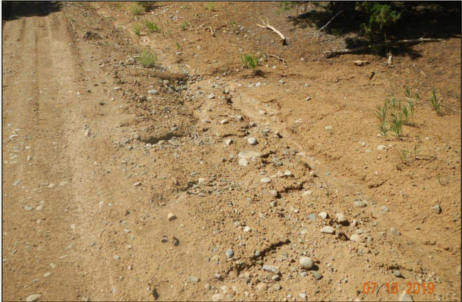
Photo 2. View of rilling and erosional down-cutting of bare soils along access road.
