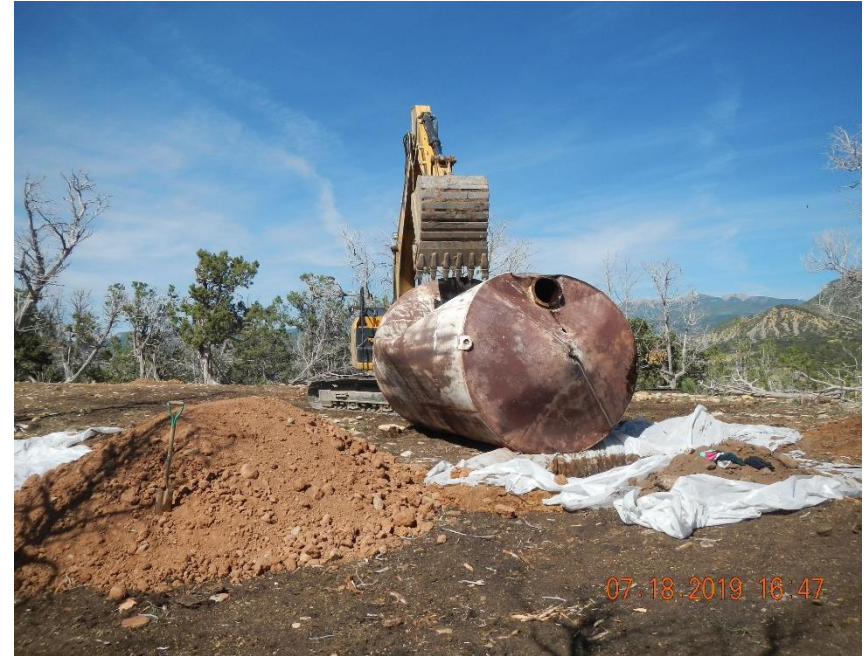
Track hoe demolishing AST.
