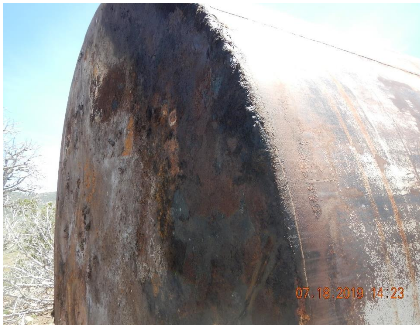
Corrosion along bottom seam of AST.
