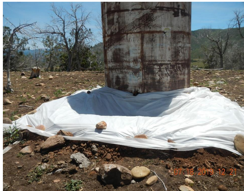
Containment area lined with plastic sheeting.
