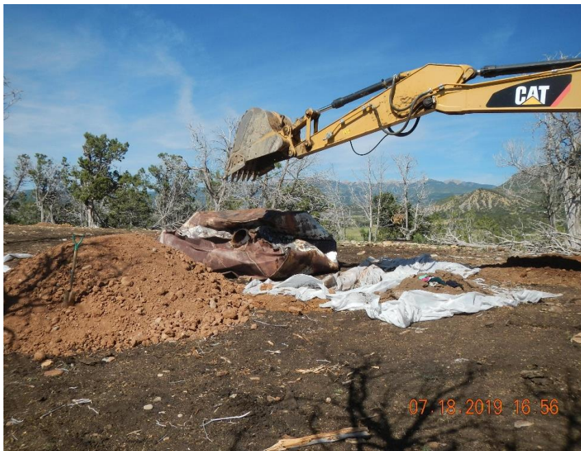
AST crushed into size to transport.
