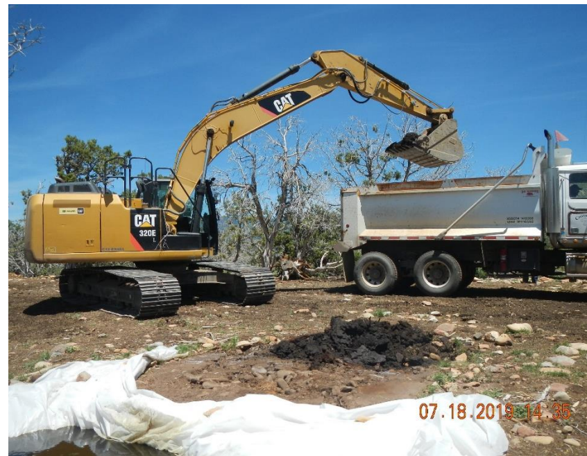
Excavating impacted material.
