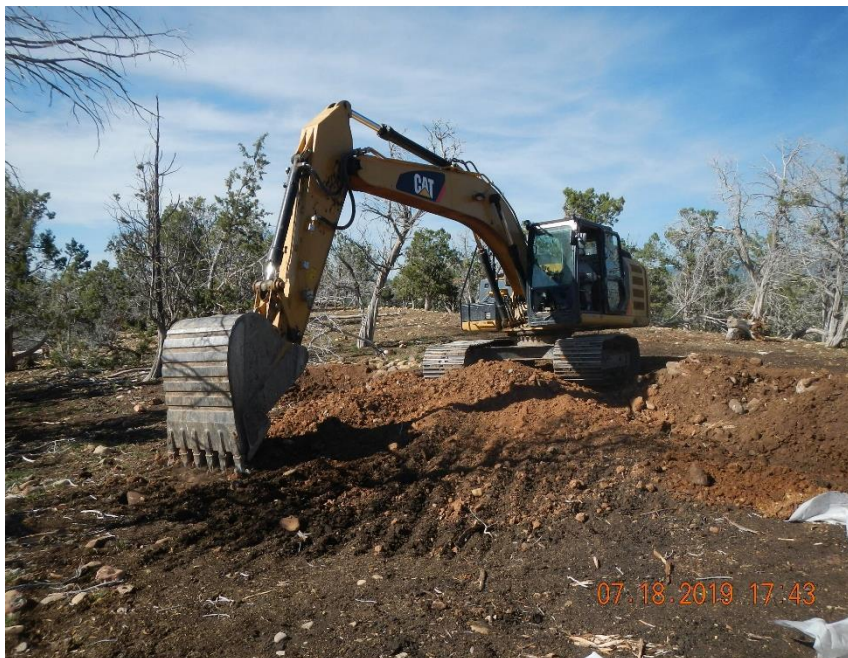
Excavated area backfilled with clean fill.
