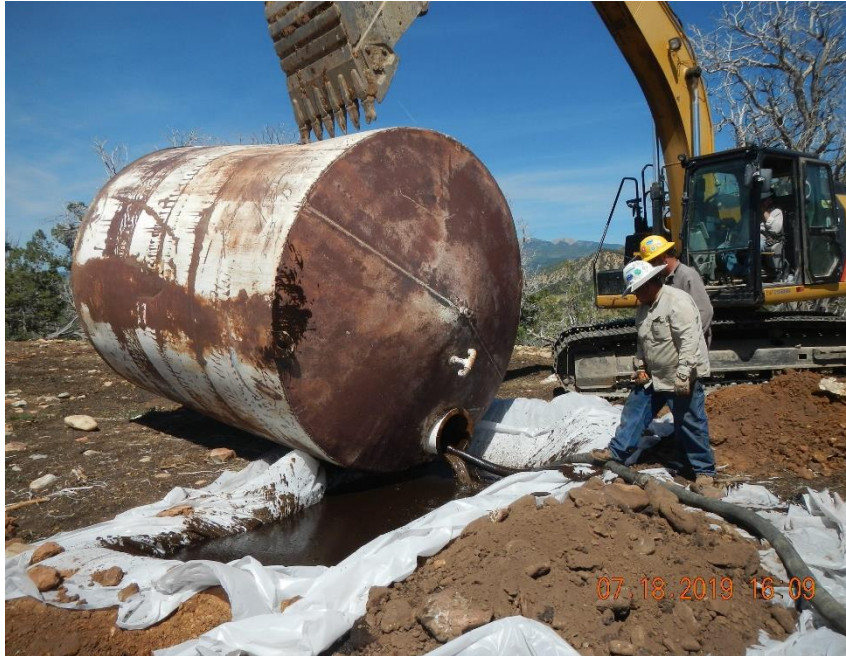
Flushing residue from AST.
