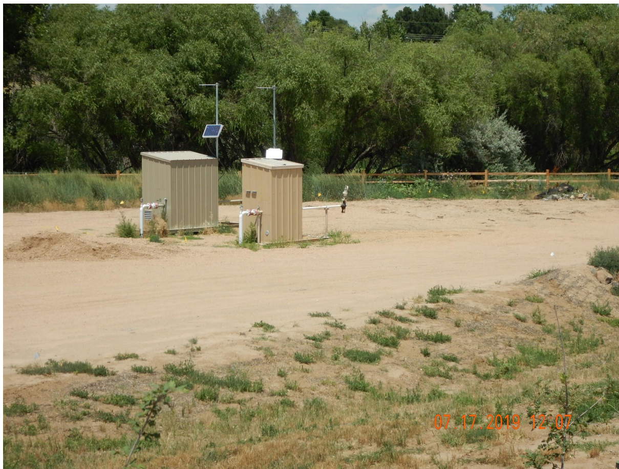
Photo 1. Photo taken of the tank battery, facing North. Photo illustrates equipment that remains at the tank battery location after plugging all associated wells. Operator shall comply with the Rule 1004 standards regarding Final Reclamation activities.
