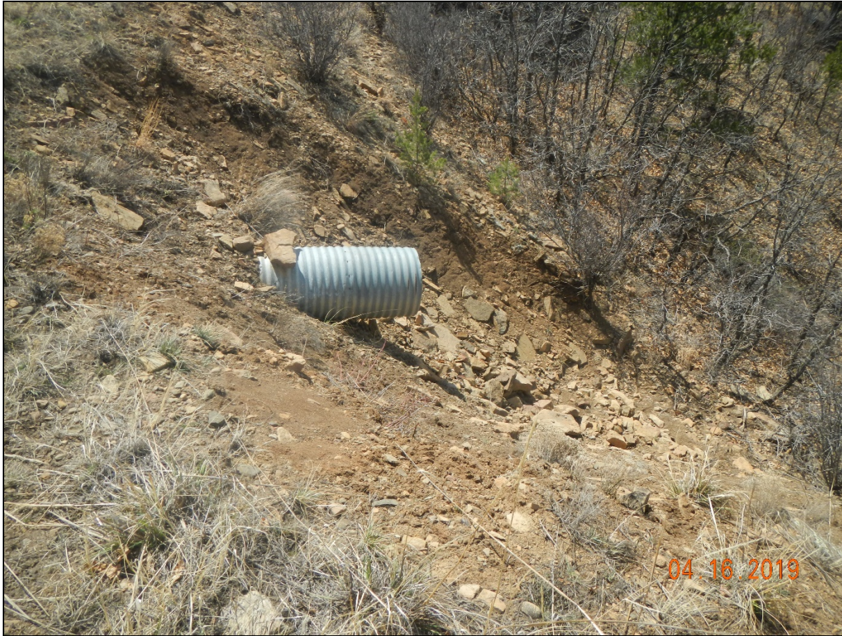
Photo 5. Culvert remains along the road. Erosion is occurring around the outlet.
