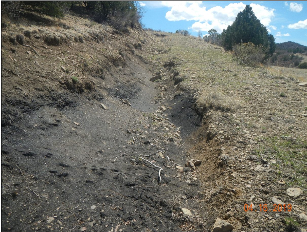
Photo 3. Photo shows erosion along the access road. Access road has not been recontoured and reclaimed.
