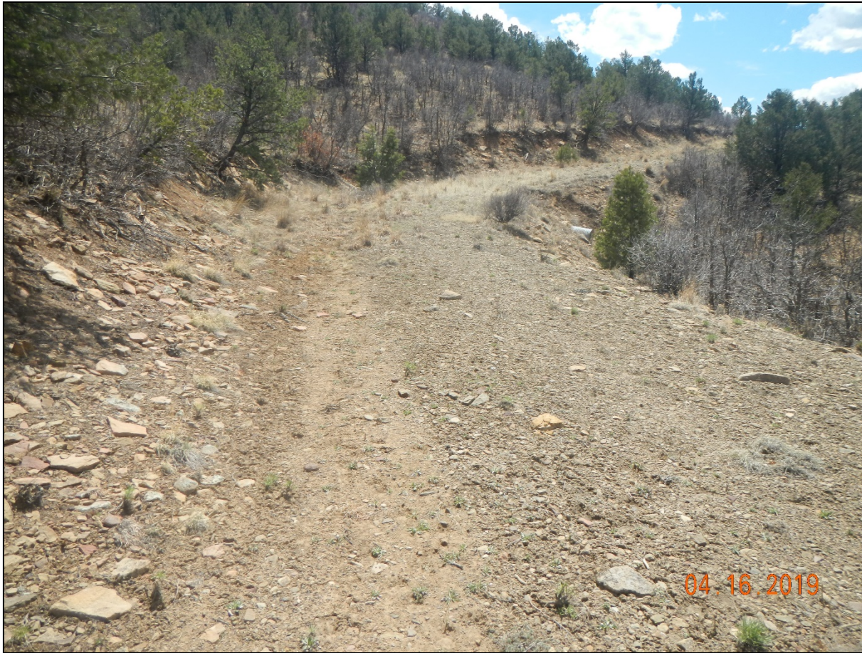
Photo 4. Further along the road. Access road has not been recontoured and reclaimed.
