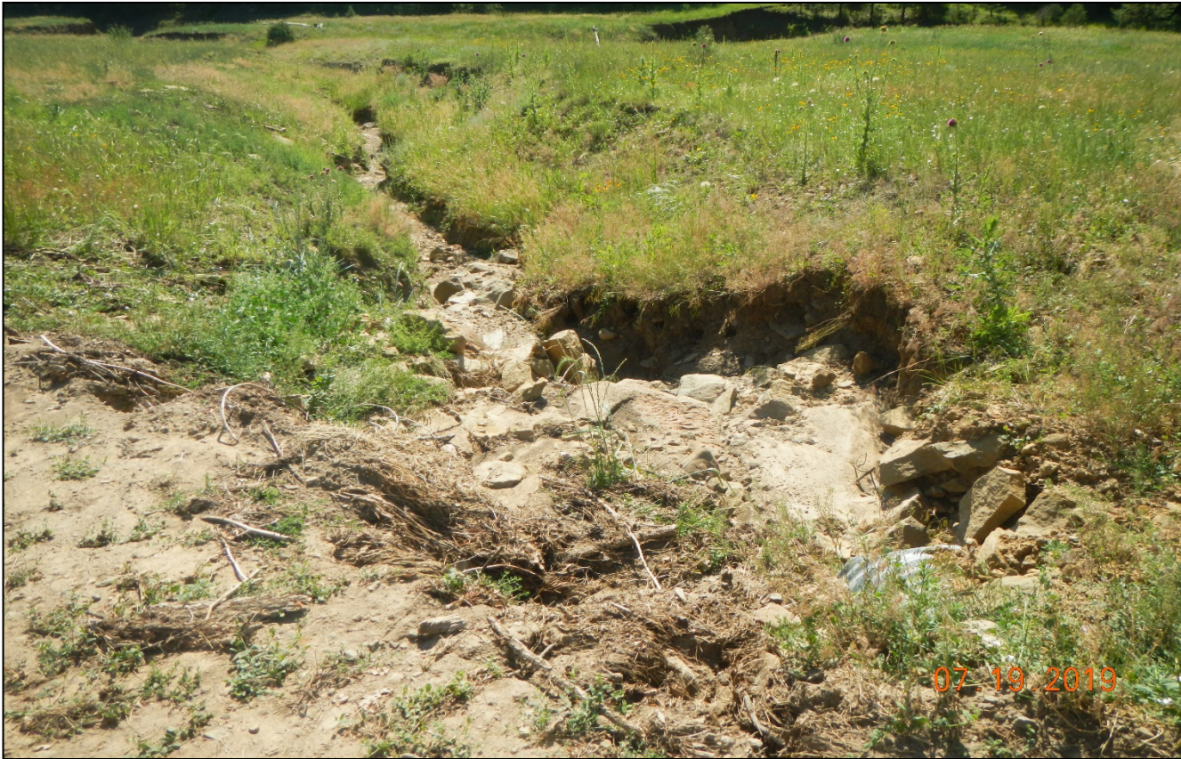
Photo 2. There is erosion occurring at the outlet culvert. No BMPs installed for outlet protection or to prevent erosion. Lat/Long:37.02425,-104.82919 Corrective action was not performed since previous inspection.
