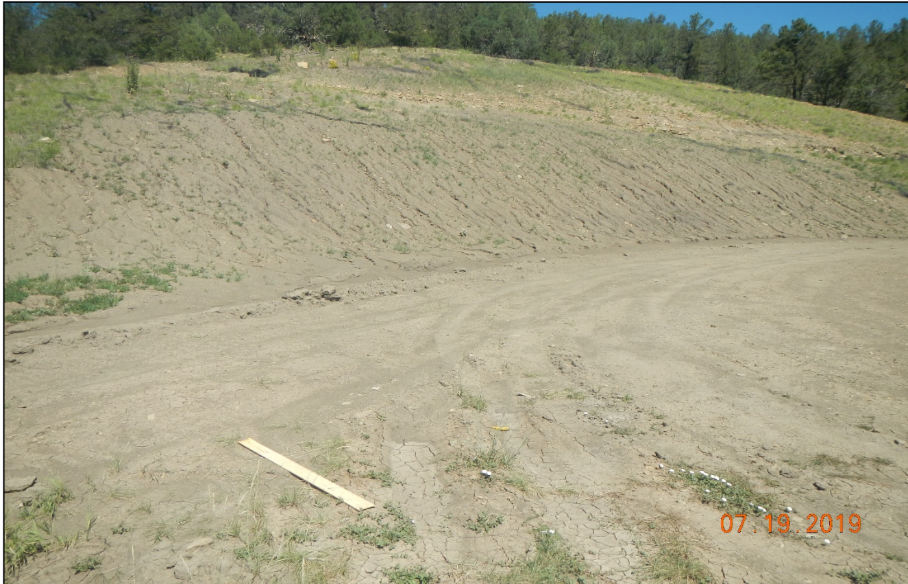
Photo 4. The cut slope is not stabilized and erosion is occurring. No vegetation is establishing. Corrective action was not performed since previous inspection.
