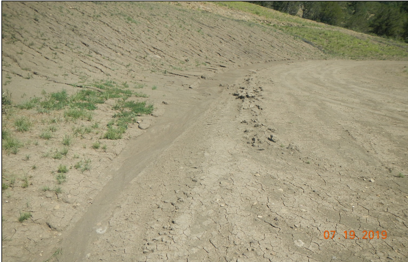
Photo 6. Sediment has already filled in the diversion ditch from erosion of the cut slope.
