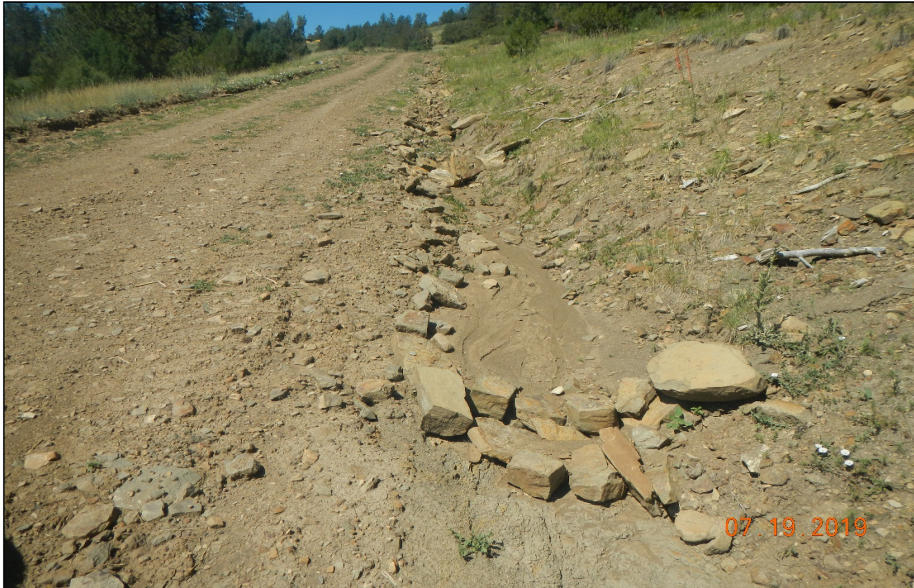
Photo 3. Rock check dams were installed along the side of the access road to the location. Sediment has filled in the check dams or stormwater is flowing around. Corrective action was not performed since previous inspection.
