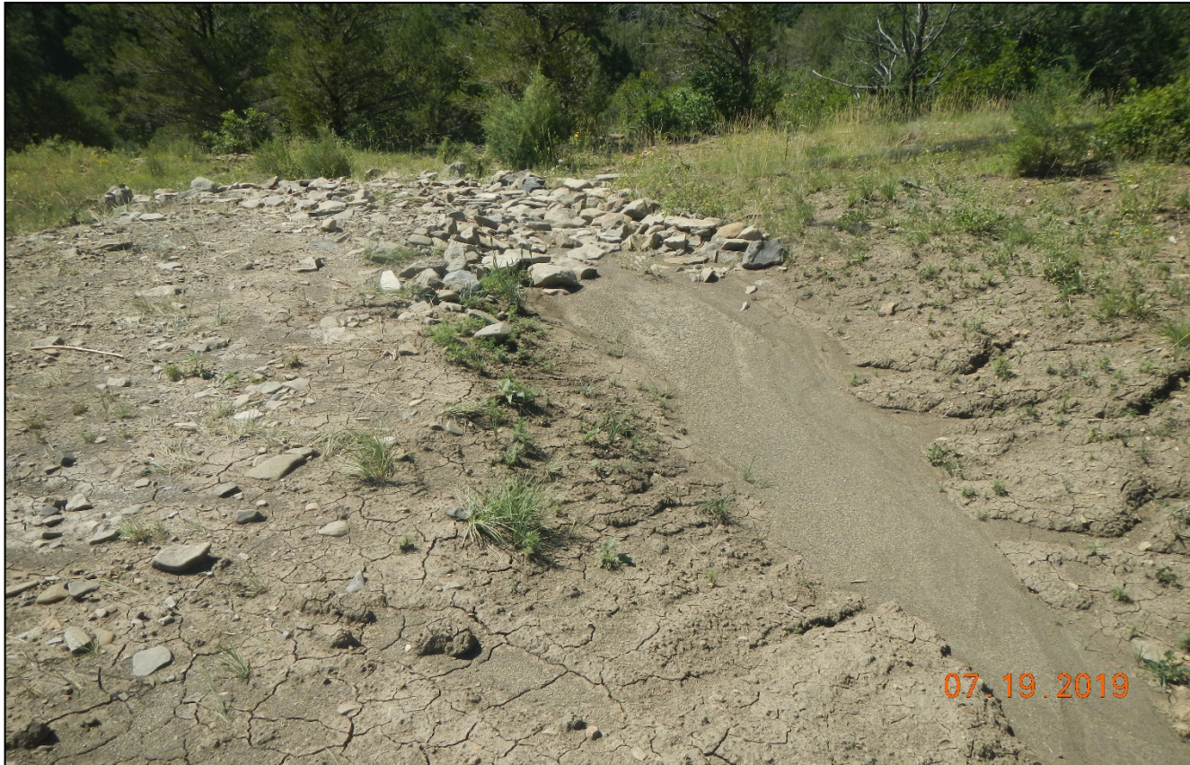
Photo 5. Rock rip/rap was installed at the end of the diversion ditch however, sediment has already filled in the diversion ditch from erosion of the cut slope.
