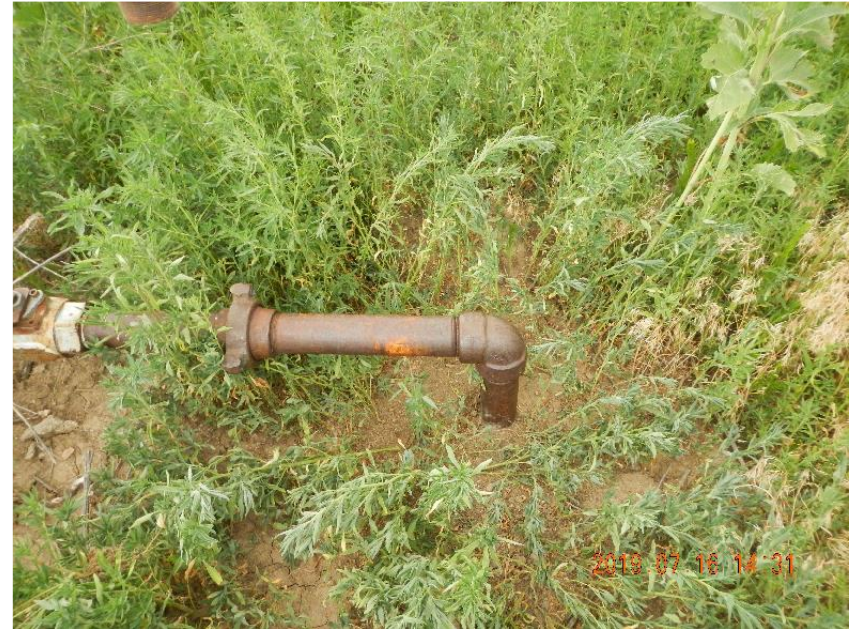
Photo 4: Connected 2" steel flow line at wellhead.
