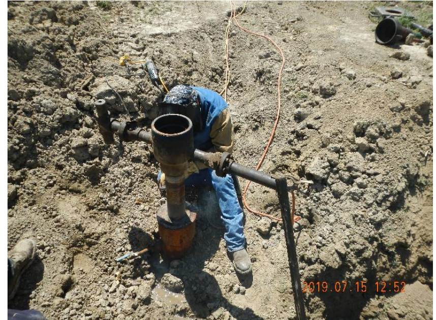
Photo 2: Setting new wellhead to be used during plugging operations.
