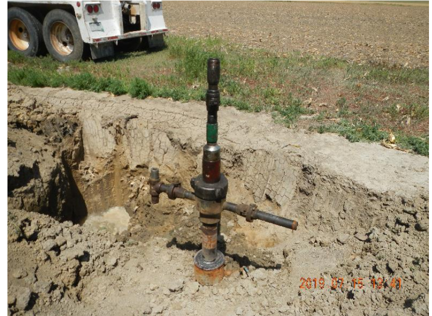
Photo 4: Wellhead completed.
