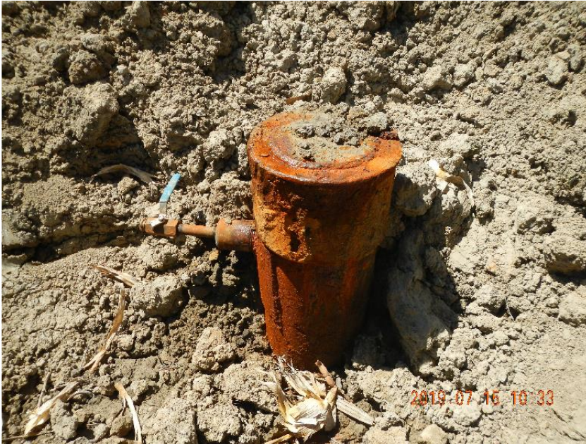
Photo 1: Vondy 3 surface casing.
