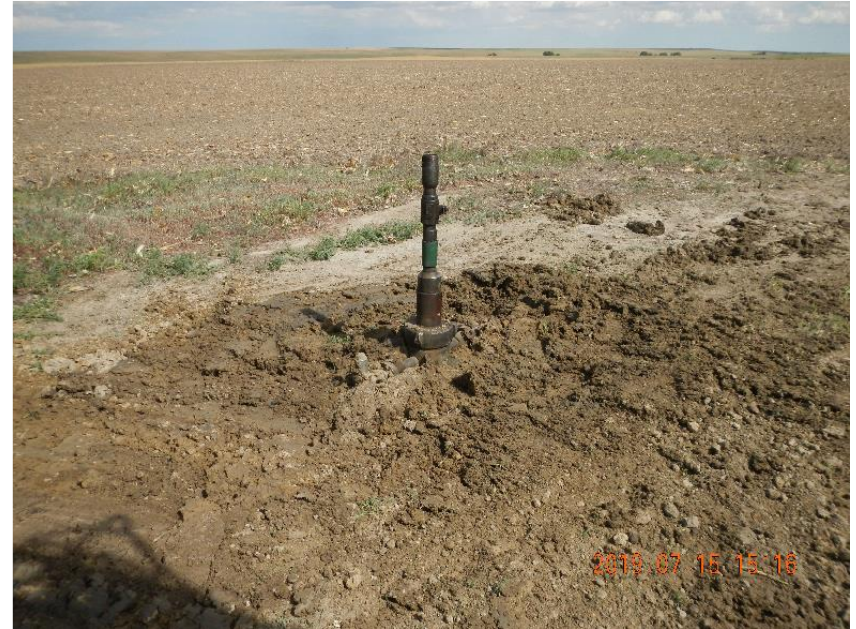
Photo 6: Area around wellhead backfilled and ready to set balance beam for rig.
