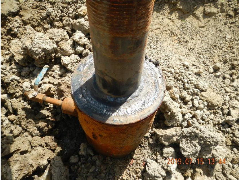
Photo 5: View of casing cap weld repairs.
