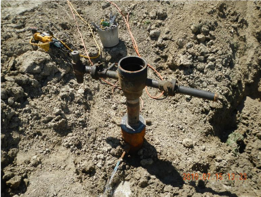
Photo 3: New wellhead welded into place. Water from well being released to allow for weld repairs.
