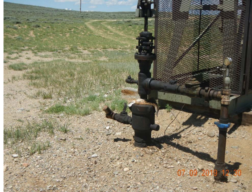
Photo 2. Rags used to stop leak at wellhead.
