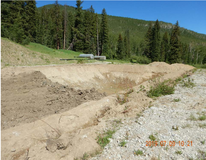
Photo #9 – View of Tepee Park CFF Pit (Facility ID #416339), looking NW. Note that pit does not have any fencing installed to prevent wildlife access.
