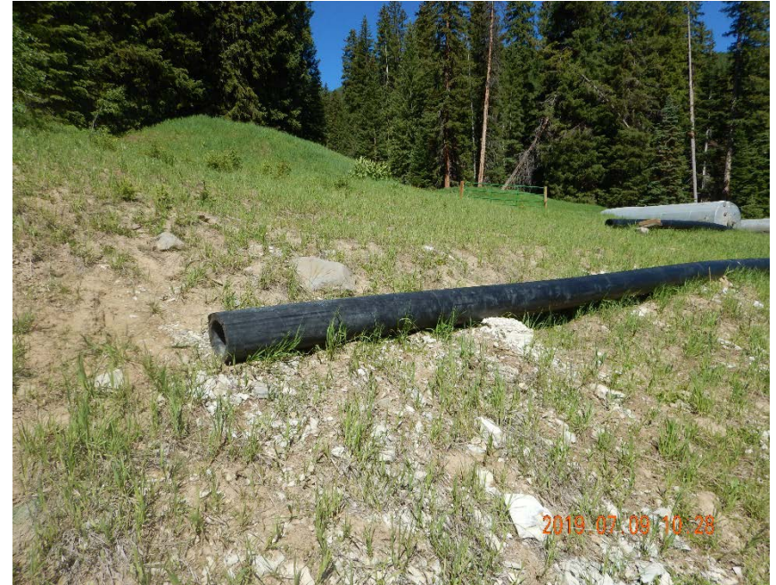
Photo #20 – Uncapped, unmarked HDPE surface flowline in Former Tank Battery area.
