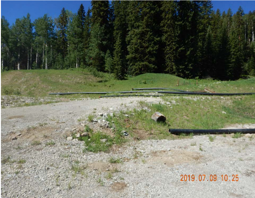
Photo #21 – Unused equipment (uncapped, unmarked HDPE surface flowlines) in Former Tank Battery area.
