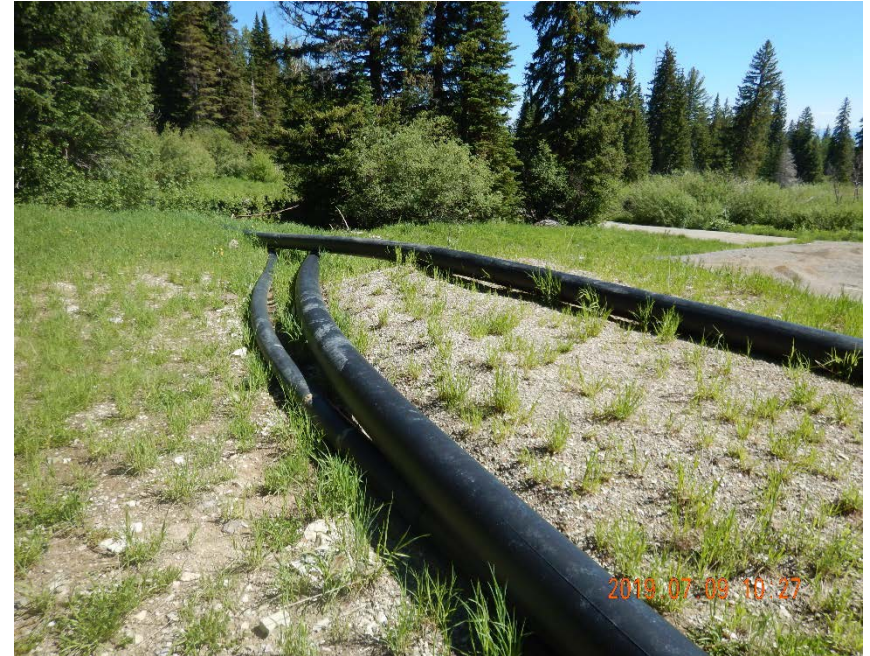
Photo #16 – Unmarked HDPE surface flowlines leading north from Former Tank Battery area.
