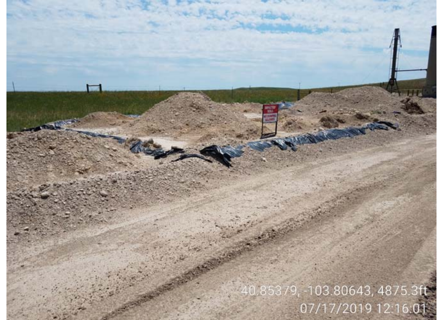
Photo 4 – Impacted material stored on location pending disposal.
