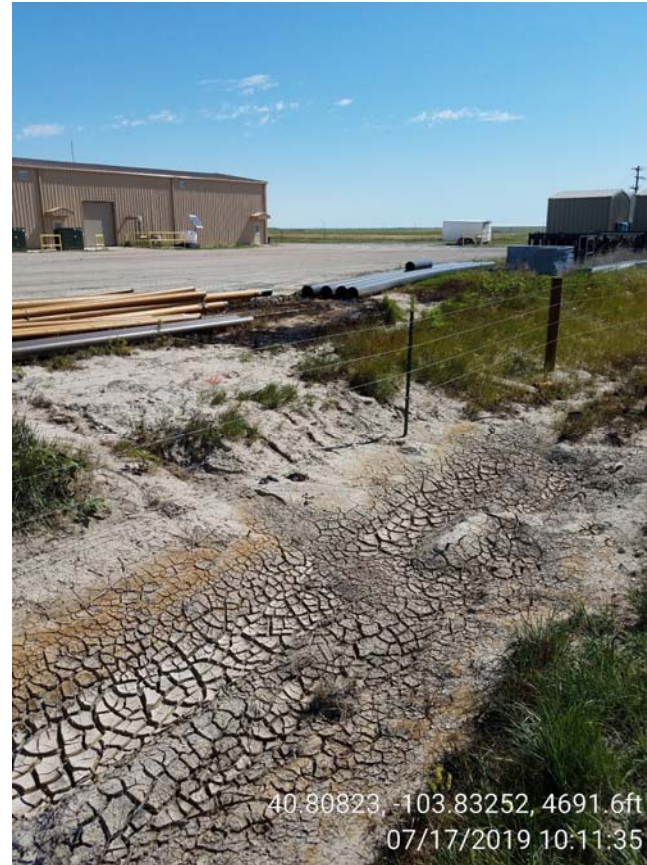
Photo 4 – Area where spilled water and oil ran off location into stormwater control ditch on southside of location.
