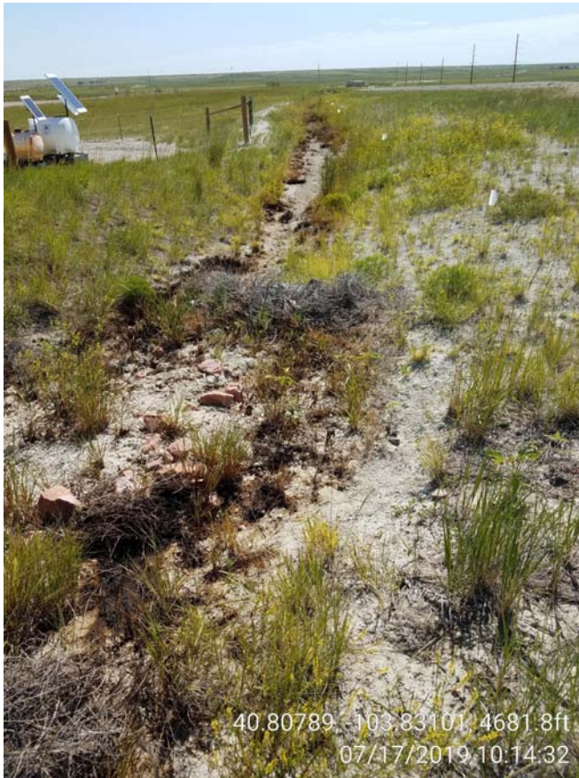
Photo 7 – Stormwater control ditch on south side of location at southeast corner of location looking east. Produced water and oil exited location near southeast corner into ditch.
