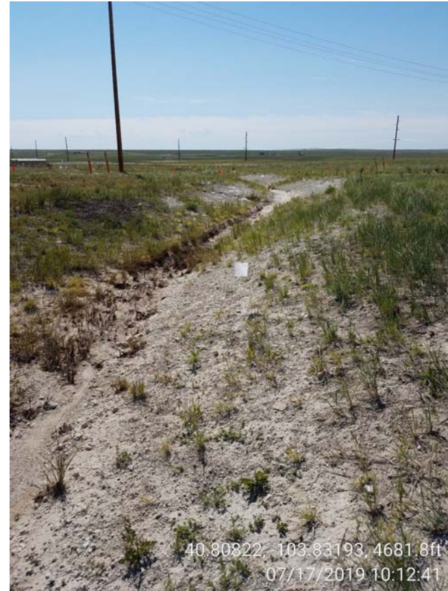
Photo 6 – Stormwater control ditch continuing east of location, impacted by produced water and oil.
