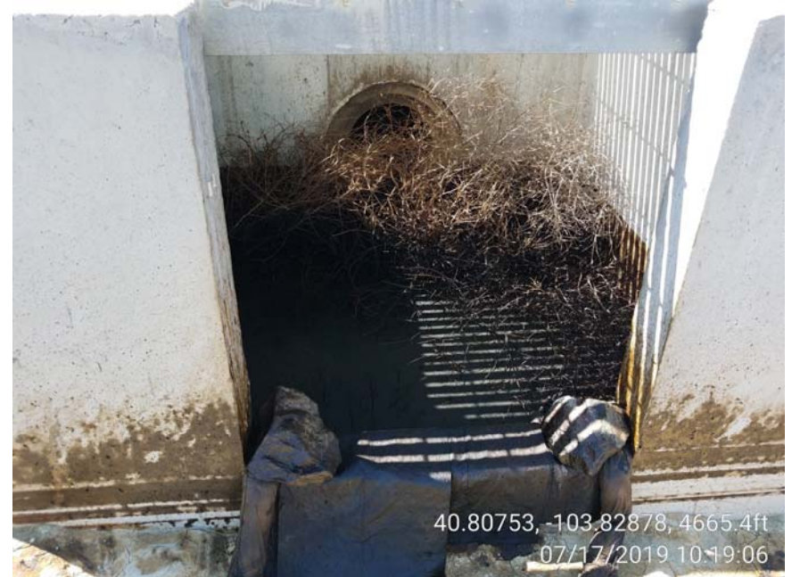
Photo 10 – Stormwater control pond outlet box impacted by oil.
