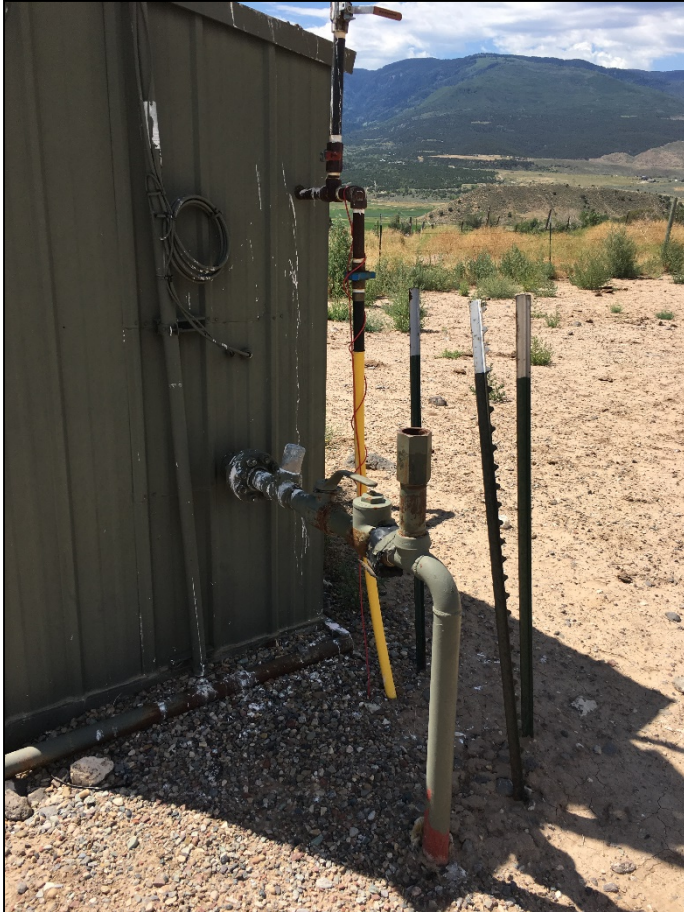
Domestic tap pictured. Yellow poly with tracer wire
