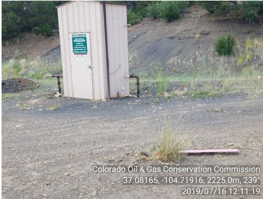
PHOTO 3: GUY LINE ANCHOR MARKER DOWN. INSTALL GUY LINE ANCHOR COMPLY WITH RULE 1003.a. CA DATE 7-31-19
