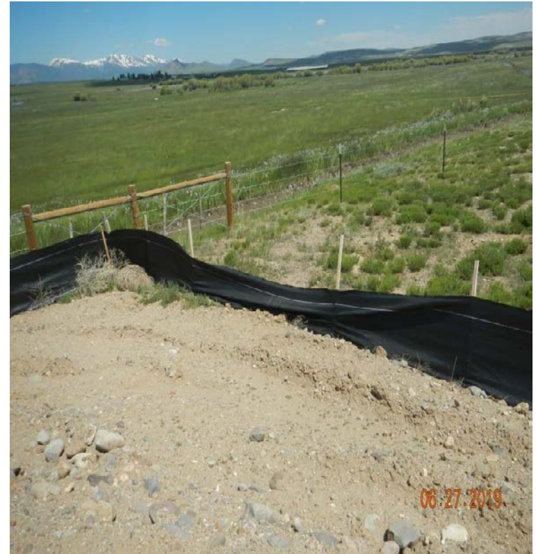
Photo#8: Silt fence failing.
