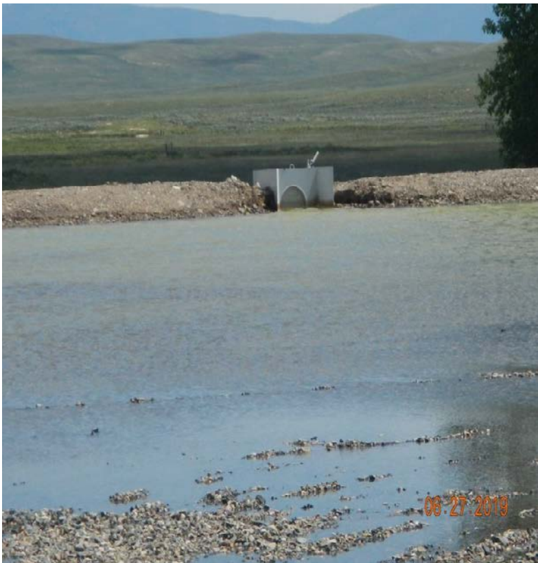
Photo#3: Weir retaining stormwater at north end of site.
