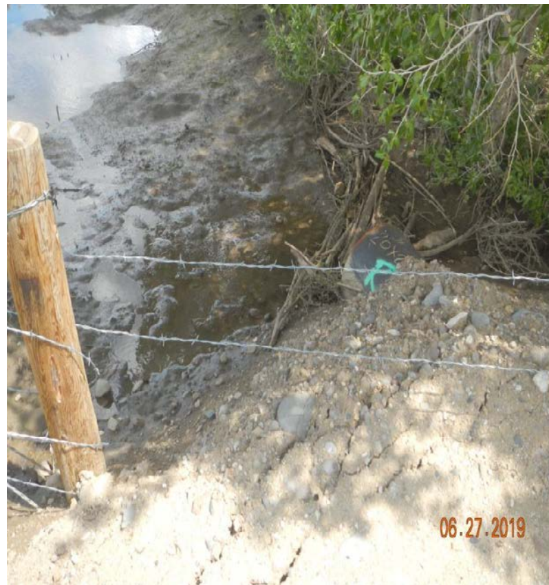
Photo#6: No sediment controls at culvert installation.
