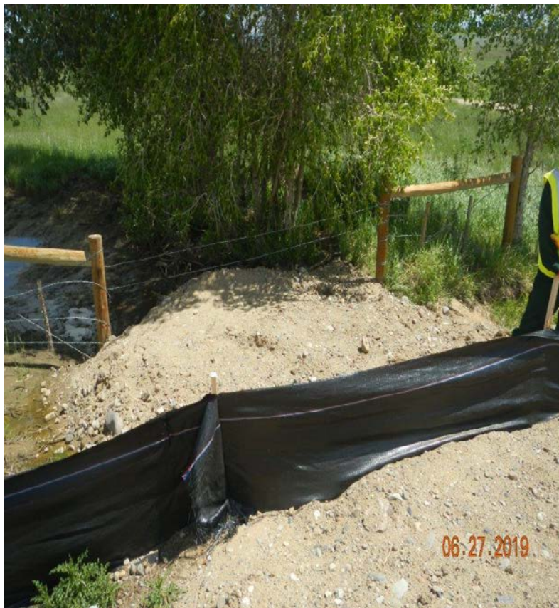
Photo#5: No sediment controls at culvert installation.
