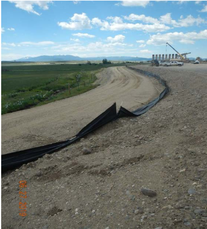
Photo#7: Silt fence failed.
