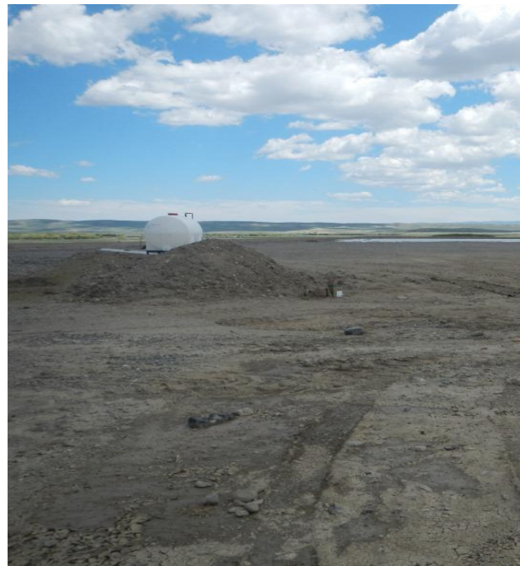
Photo#4: Unconsolidated stockpile with no BMPs employed.
