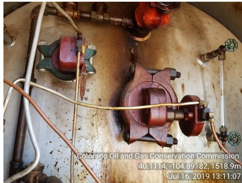
Photo 18 Mechanical issue: Piping on separator
