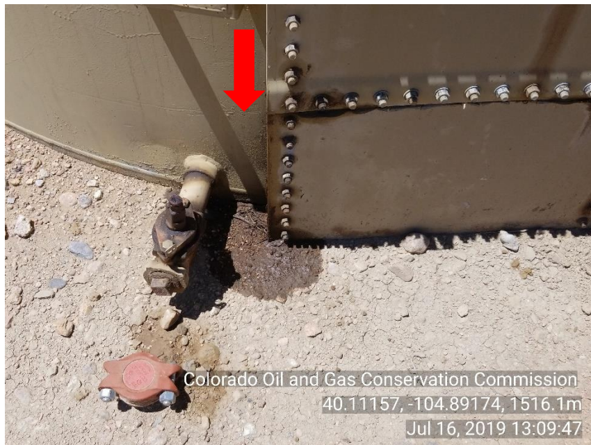
Photo 13 stained soil around load line of crude oil tank
