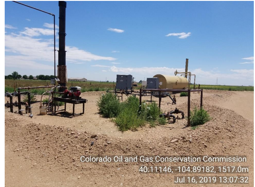
Photo 8 sep/meter runs and ECD equipment not running. Weeds around equipment.
