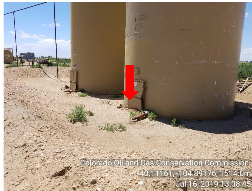
Photo 12 Stained soil around inspection hatch of Crude oil tank.
