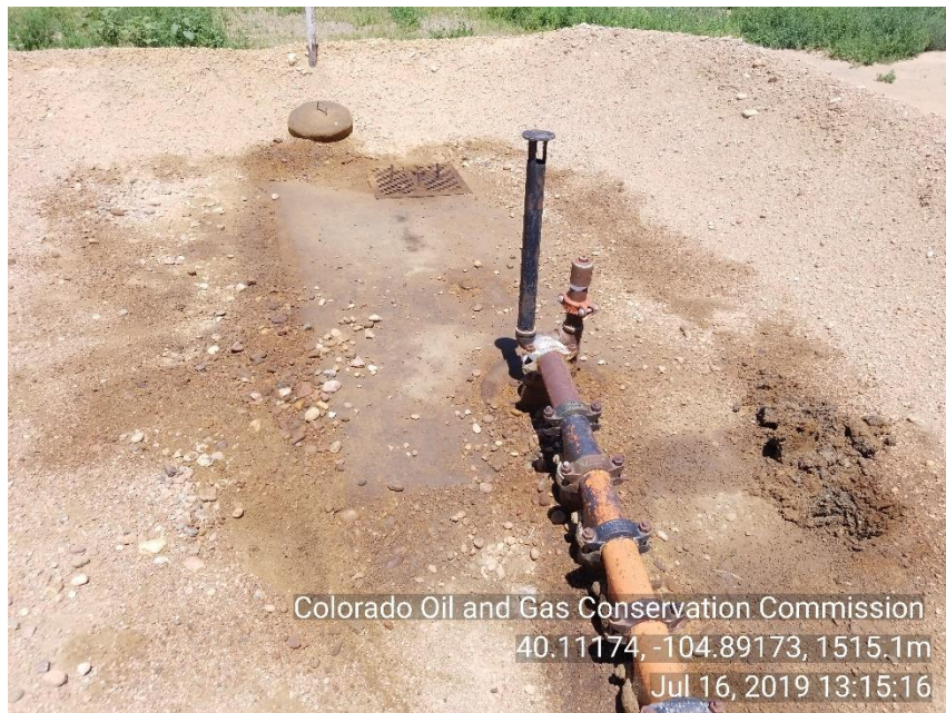
Photo 11 Produced water tank. Appears tank overflowed inside containment. Spill
