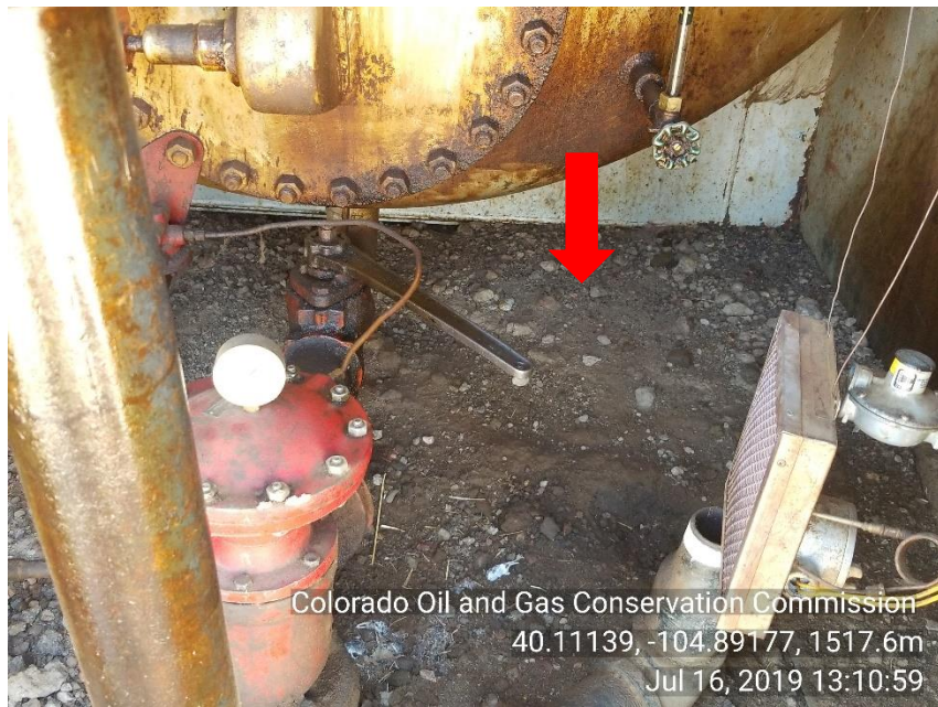
Photo 17 stained soil inside Separator house. Mechanical Issue: Piping on separator.
