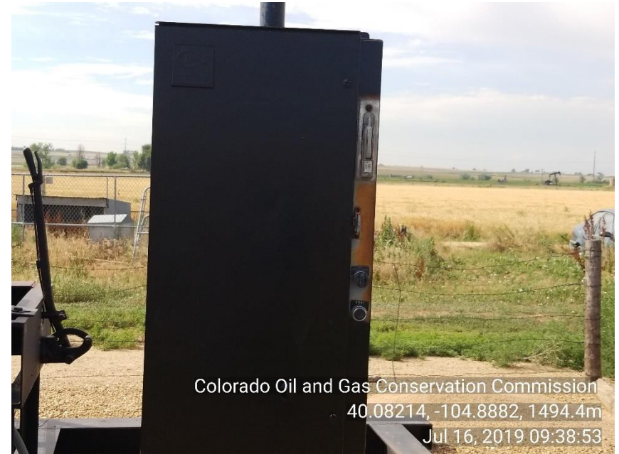
Photo 8 Breaker box at PU is in the off position.
