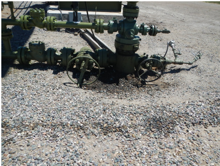
17) Housekeeping – impacted material around wellhead
