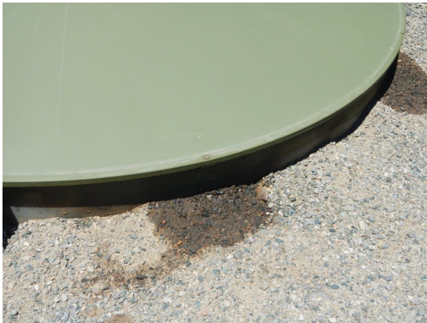
4) Actively leaking PBV, no labels or placarss
