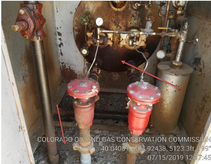
Pic 5 stained soil/possible leak inside separator house
