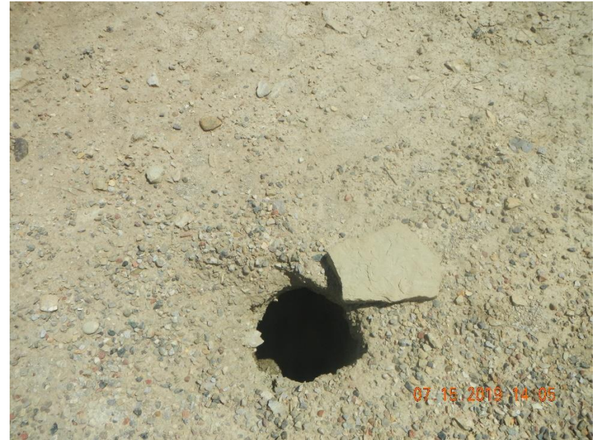
Open hole next to well head.
